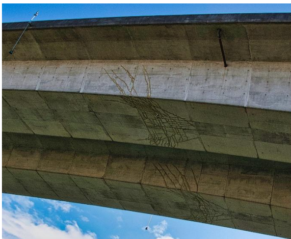
Figure 5. West Seattle Bridge (source: https://www.westsideseattle.com )
