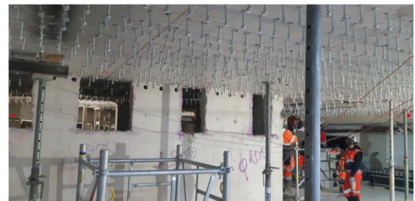
Figure 12. Example of the use of Hilti HCC-HUS4 concrete screw connectors on the underside of a slab.
