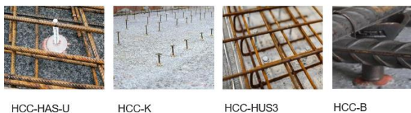
Figure 3. Installation of Hilti HCC shear connectors with and without overlying reinforcement layer
