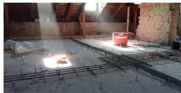
Figure 13. Attic reinforcement in a residential building with Hilti HCC-HUS4 concrete screw connectors
