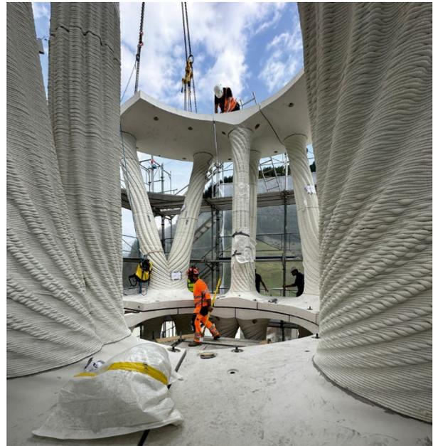
**Figure 3. 3DPC structure assembly (level 3).**
