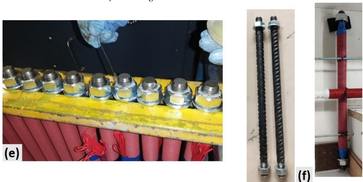
Figure 8. e) Resin application for the connection to rebar f) Prepared headed bars.
