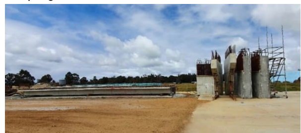
Figure 14. Bridge 0235A storage of all precast elements
