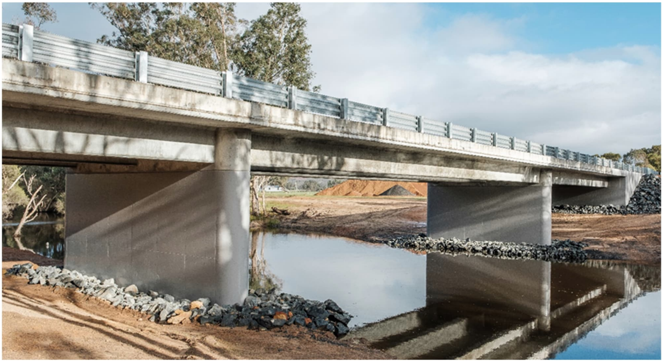
Figure 5. Bridge 0270A after completion
