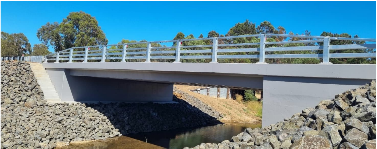
Figure 15. Bridge 0235A installed
