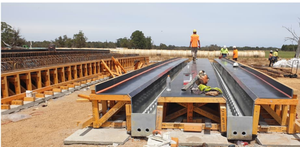
Figure 1. Simple formwork set-up for 18 m span beams
