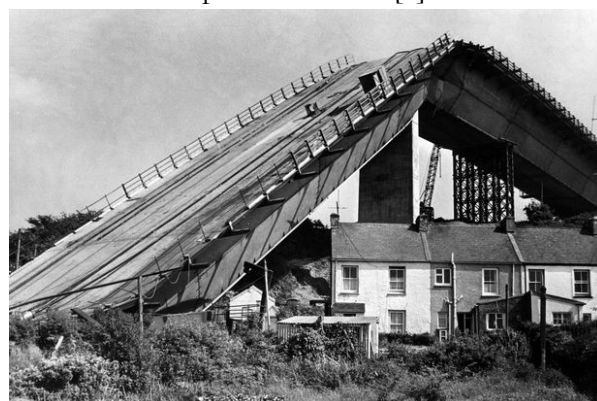
Figure 1. Cleddau bridge collapse. June 2, 1970
