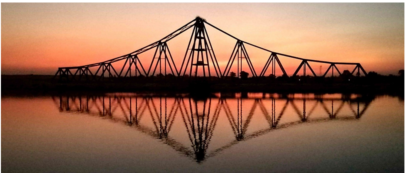
Figure 17. Existing bridge, prior to be upgraded, parked at the West side
