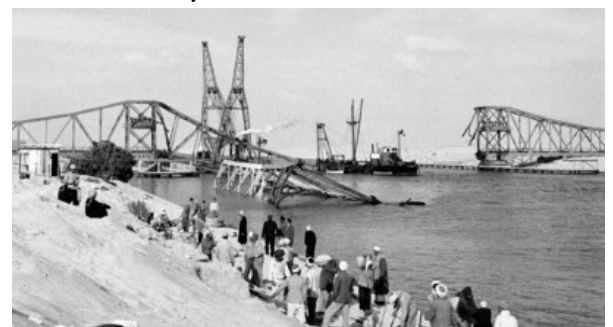
Figure 6. Removing of bridge in January 1957
