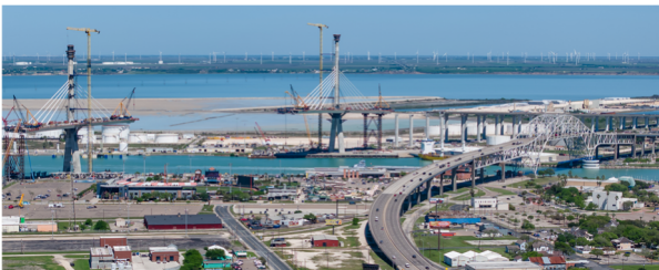
Figure 1. General view of the shipping canal with the old and new bridge during construction (Sep 2023).
