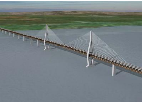
Figure 10. Third Orinoco bridge.
