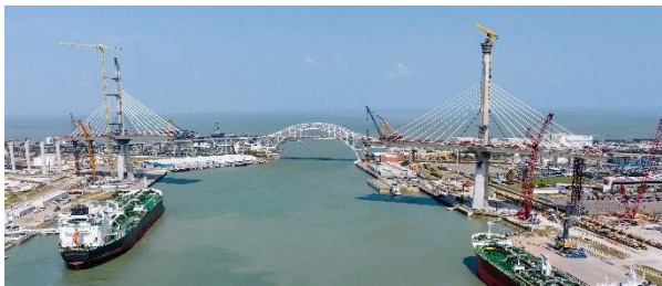
Figure 1. General view of the shipping canal with the old and new bridge during construction (April 2024).
