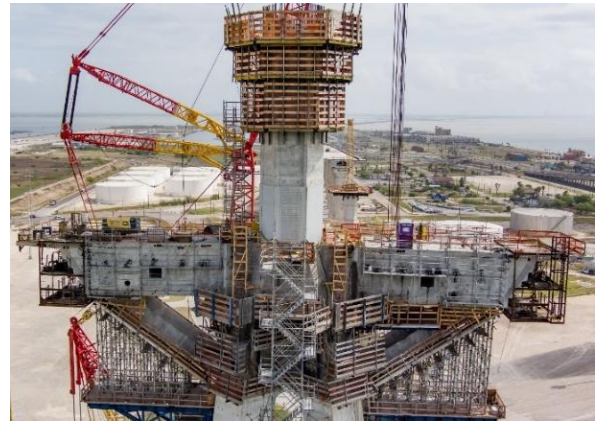
Figure 6. Tower table and upper tower first few lifts
