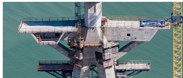
Figure 13. Dry-runs allowed for any minor misalignment of the PT ducts, across the joint, to be resolved in advance of segment erection.
