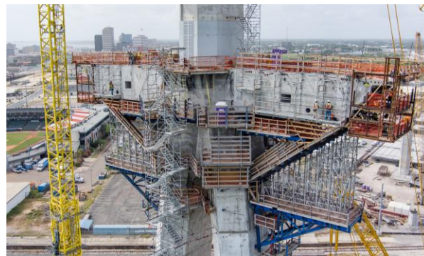
Figure 12. Construction of the tower table.
