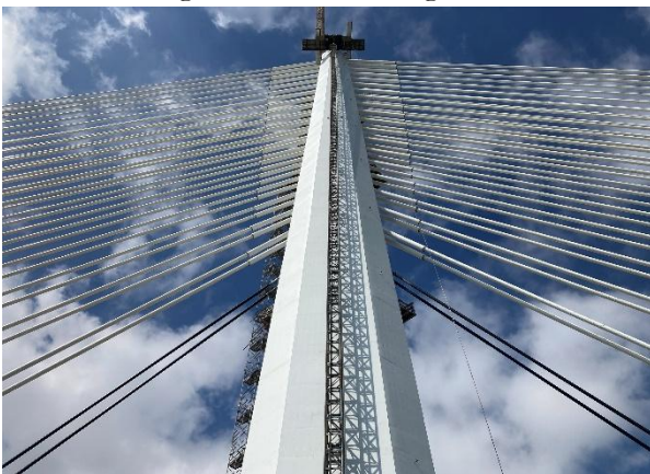
Figure 24. Stay cable forces were measured and used for Final Acceptance according to PTI [6].
