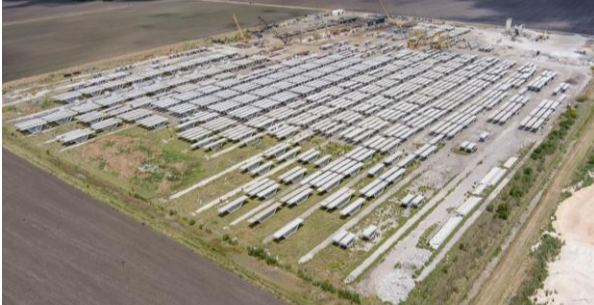
Figure 4. Precast components were stored in the yard and transported 35 km (22 miles) to the erection site using specialised haulers.
