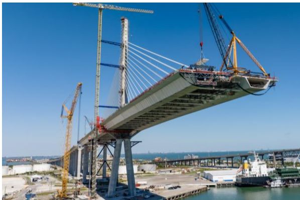
Figure 11. The stay cable anchor boxes were cast into the upper tower and used as permanent formwork.
