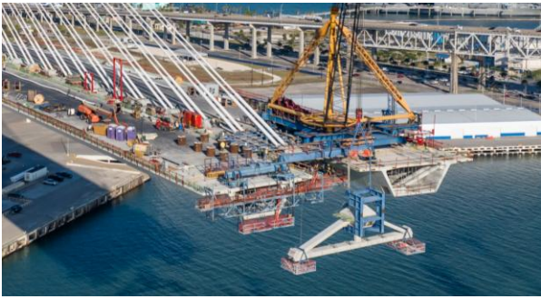
Figure 16. Delta frame installation process.
