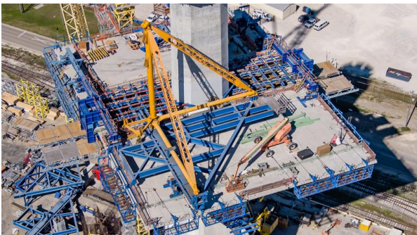
Figure 14. Main span derrick installation.
