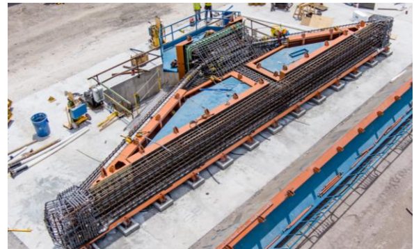
Figure 5. There were two molds for the delta frames.
