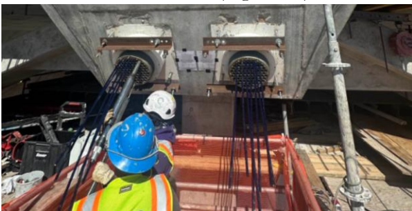
Figure 17. Epoxy coated 7-wire strand was installed and restressed using a mono-strand. Stays cables varied from 70 strands to 121 strands.
