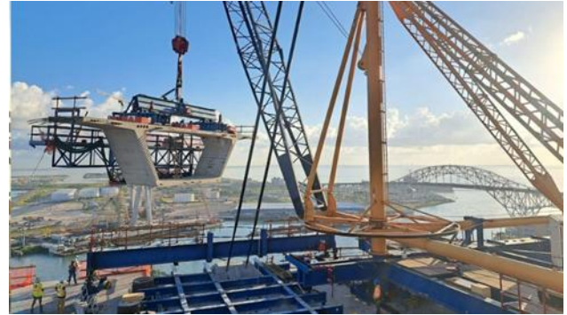
Figure 15. Segment erection with manipulator and stressing platform.
