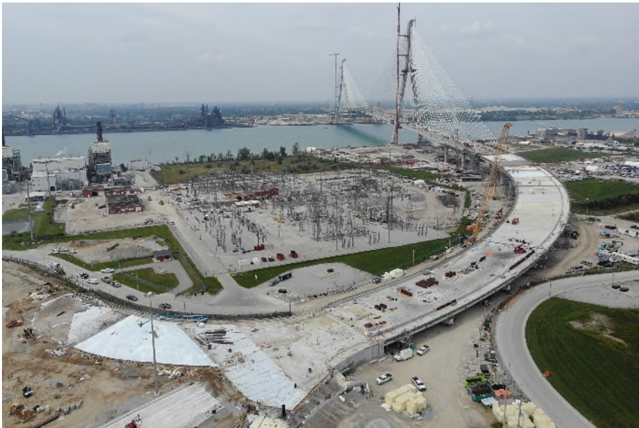
Figure 1. Canadian approach viaduct
