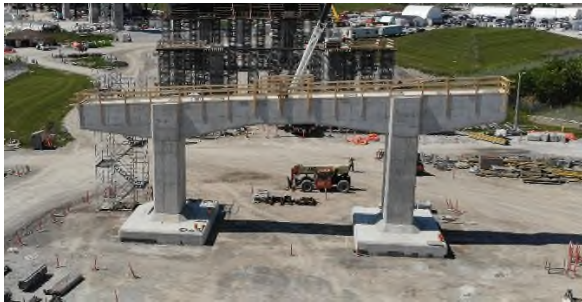
Figure 5. Viaduct substructure
