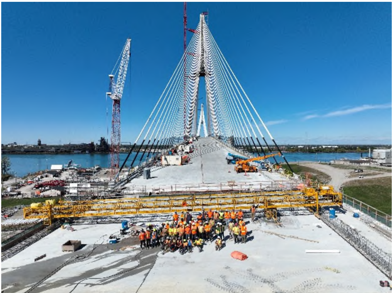
Figure 12. Erection team at Canadian approach
