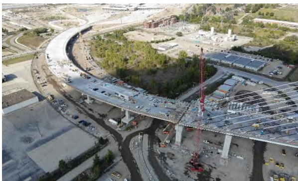
Figure 2. US approach viaduct
