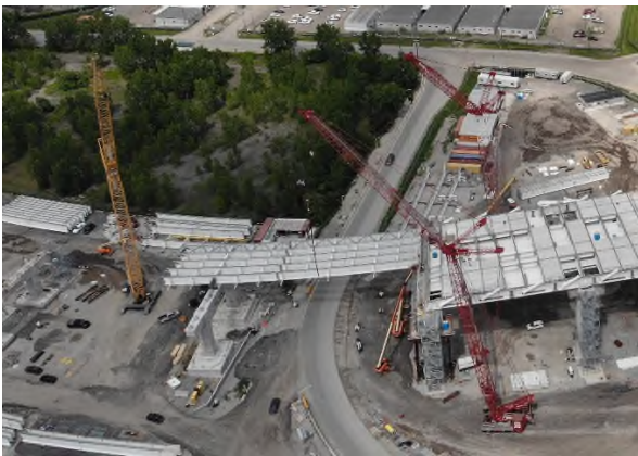
Figure 8. US viaduct erection
