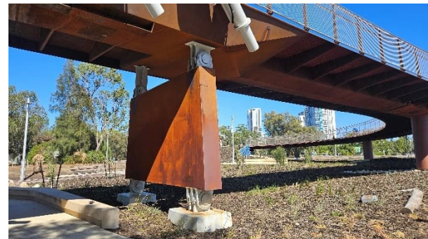
Figure 7. Pier 3 and Deck Transition of Point Fraser Bridge
