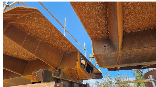
Figure 11. Stabbing guides to align deck segments
