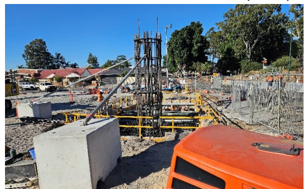
Figure 16. Anchor bars with templates installed in pile cap
