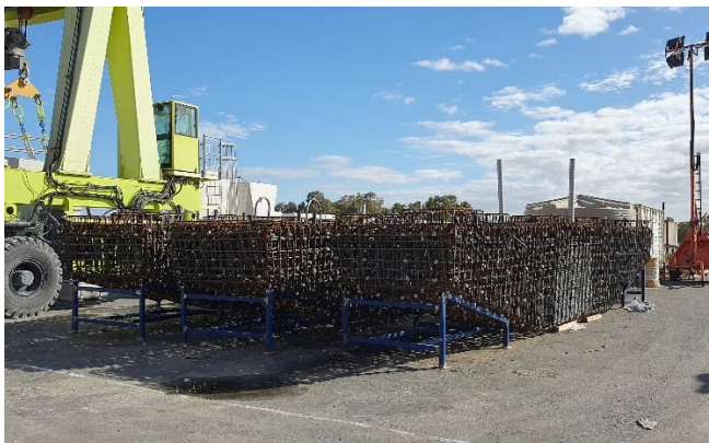
Figure 19. Pre-manufactured reinforcement cages for headstocks and viaducts
