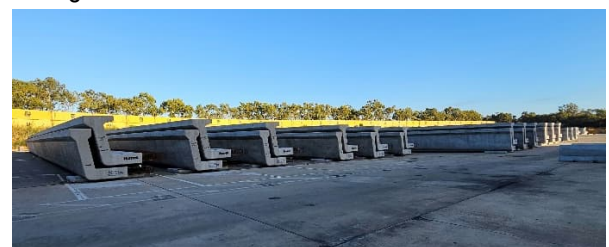
Figure 7. Stacking of L-beams in the stockyard
