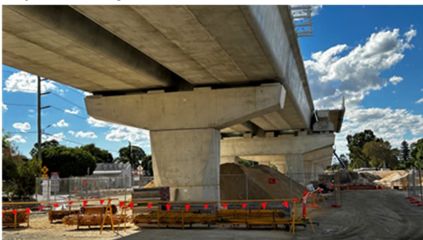
Figure 21. Viaduct partially completed
