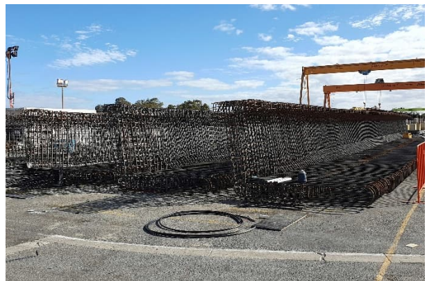
Figure 19. Pre-manufactured reinforcement cages for headstocks and viaducts
