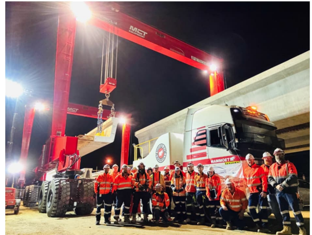
Figure 18. Gantry cranes for L-beam installation
