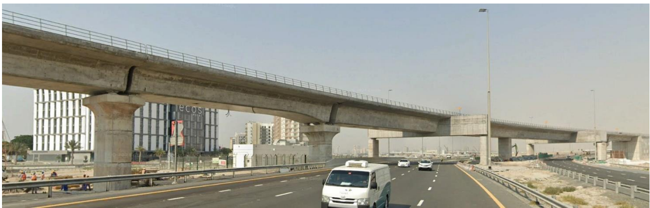
Figure 9. Viaduct 12+680. Last structural units with the portal frames
