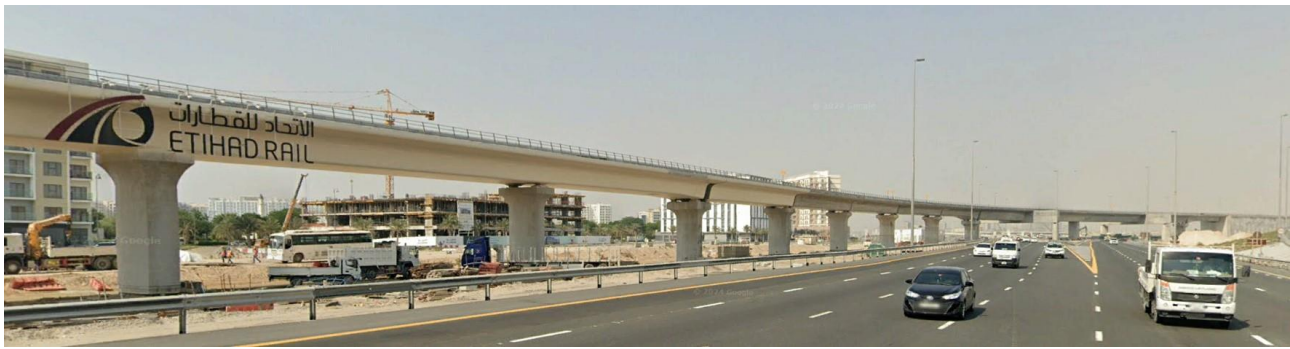
Figure 6. Viaduct 12+680. First structural units.
