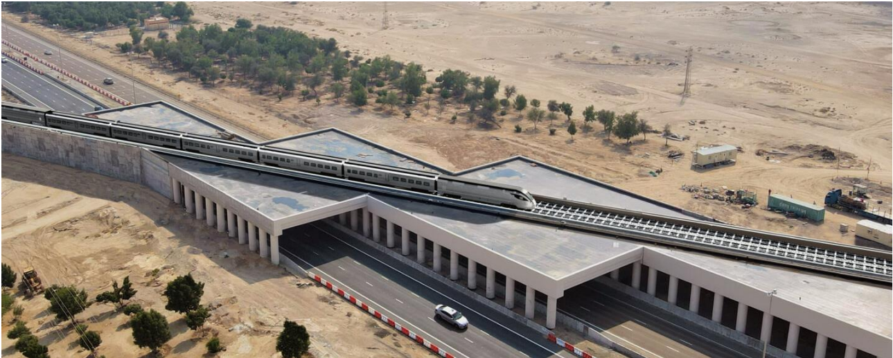
Figure 4. Bridge 13+796 in Segment 2B.
