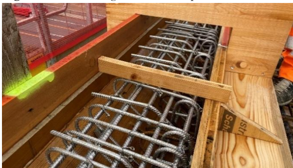
Figure 25. Steel reinforcement of the deck slab edge
