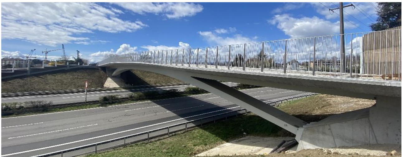
Figure 29. Main structure completed
