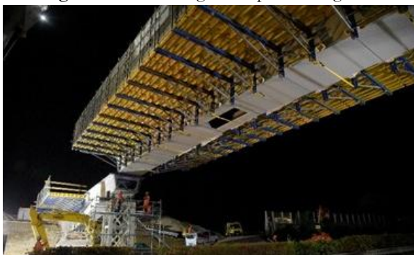
Figure 23. Installation of the steel deck of the main span
