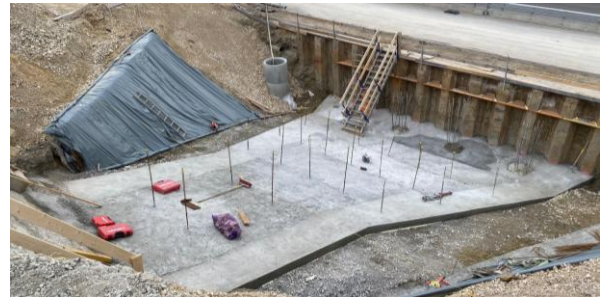
Figure 17. Sheet pile enclosure, excavation and lean concrete execution (phase III)
