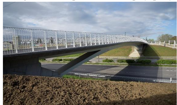
Figure 28. Main structure completed
