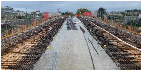
Figure 24. Concreting of the central part of the deck slab
