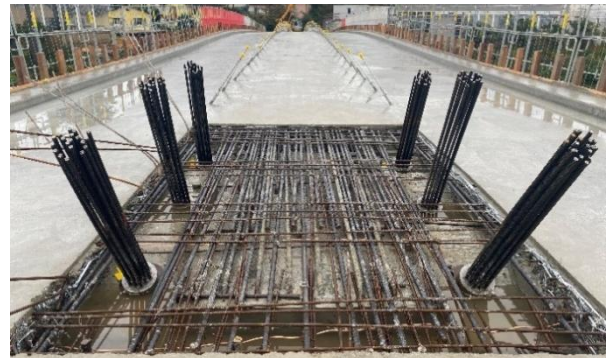
Figure 27. Prestressing cable tensioning completion
