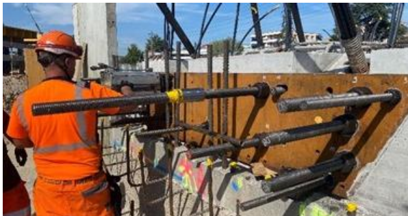
Figure 22. Tensioning of the prestressing bars
