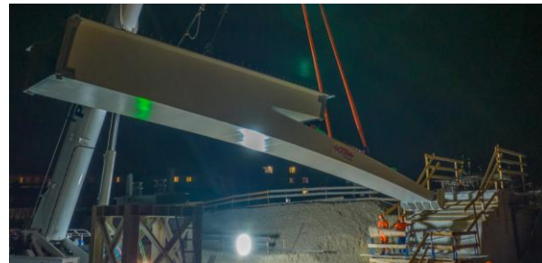
Figure 20. Installation of one pier + deck node
