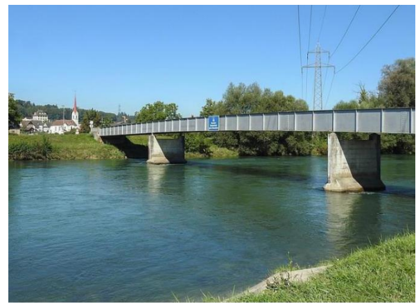
Figure 1. Reuss bridge near Mühlau, Switzerland (Source www.schweizmobil.ch , January 2022).
