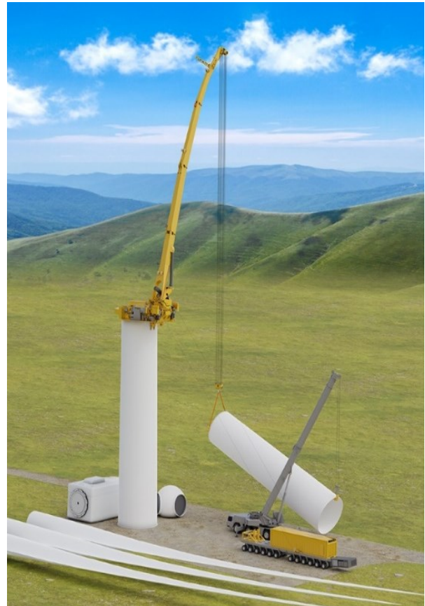
Figura 8. Liftra Crane LT1500
