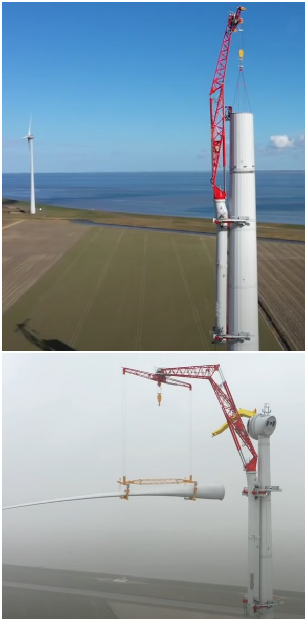
Figura 5. Climbing Crane LCC140
