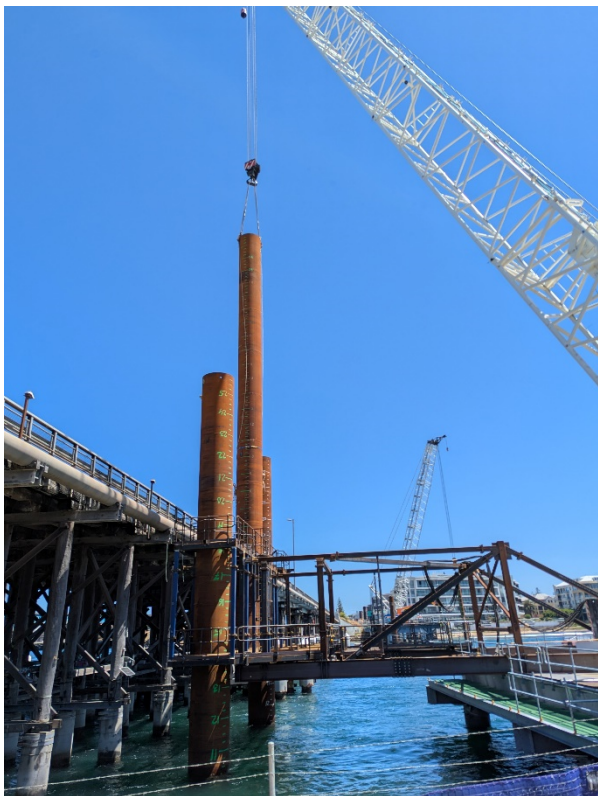
Figure 19. Installation of piles near the existing bridge, from temporary platform.
