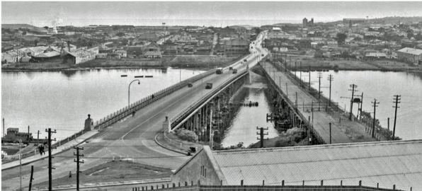
Figure 2. Current Fremantle crossing just after opening, 1940
