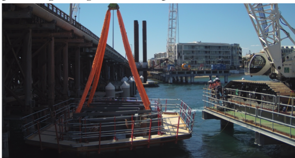
Figure 18. Precast pile-cap shell, February 2025.
