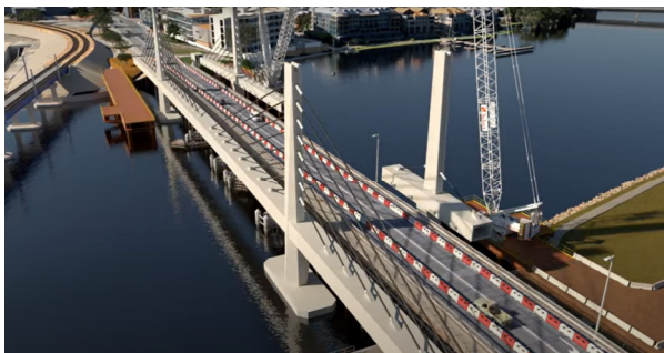
Figure 8. Edge box construction while keeping the existing bridge open.
