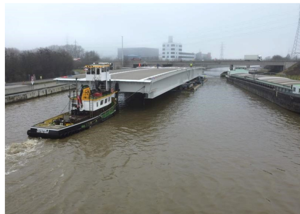
Figure 1: Sarens twin barges Karel-Victor transport 2.200 tons mobile deck from Bumas to Kluizendok.
