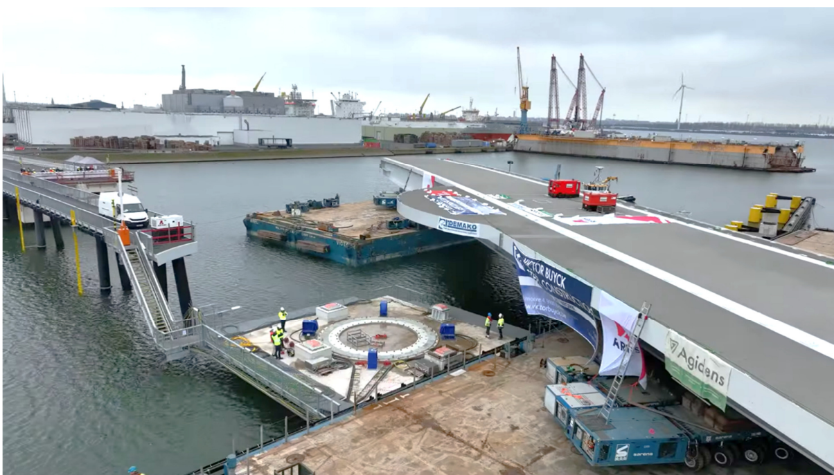
Figure 14: Detail of the final concrete foundation in between Louis and Karel-Victor barges right before reaching the final bridge position.
