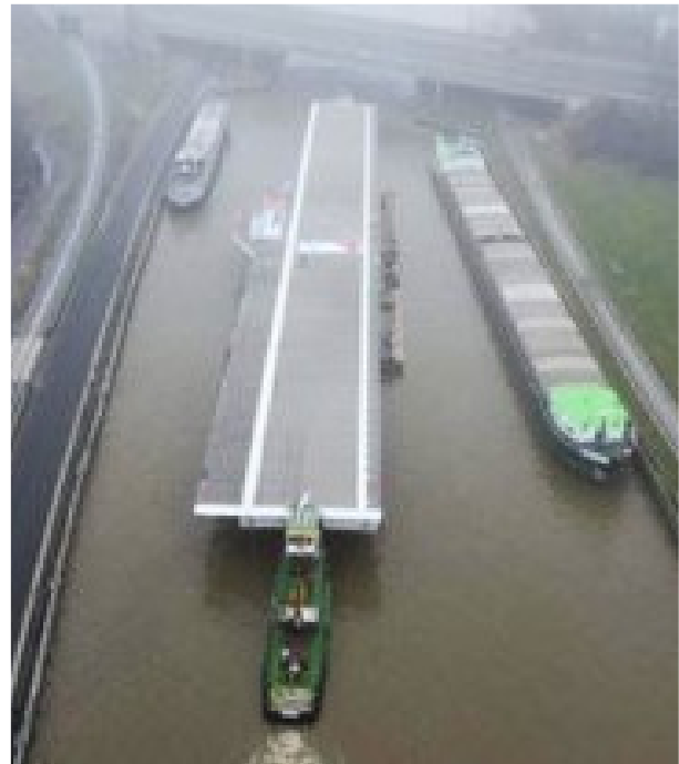
Figure 2: Mobile deck approaching to the lowest canal bridge that had to be crossed.
