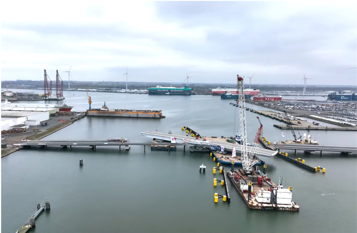
Figure 15: Side view of the mobile deck and carousel right over the final concrete foundation.
