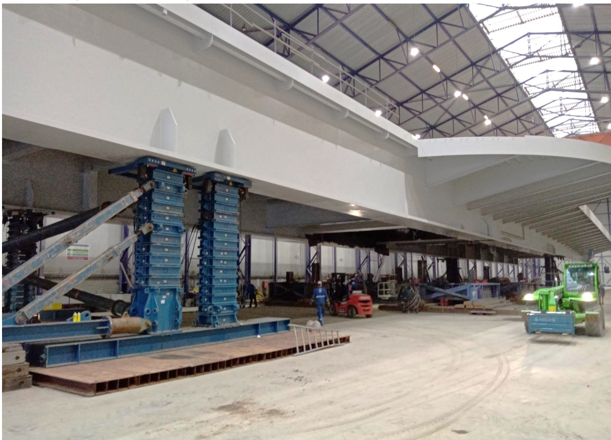
Figure 4: 130m mobile deck completed at Wondelgem fabrication workshop in Ghent during the 2,5m jacking with 4 climbing towers of 2x450 tons to attach the carousel crown below it.
