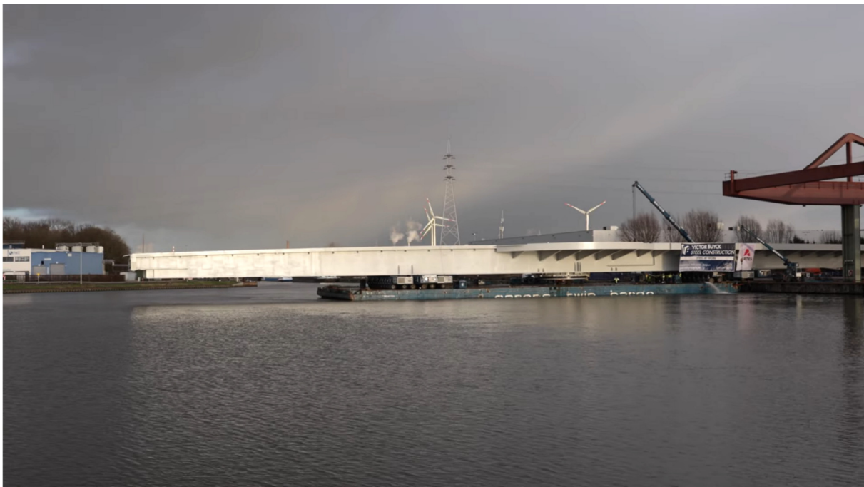
Figure 6: Mobile deck and carousel at the end of the load out on Karel-Victor twin barges at the yard of client fabrication workshop in Wondelgem.
