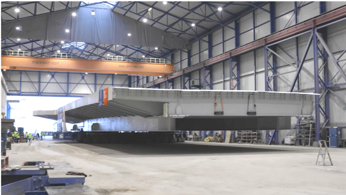
Figure 5: Mobile deck and carousel supported on SPMTs driving out the fabrication workshop.
