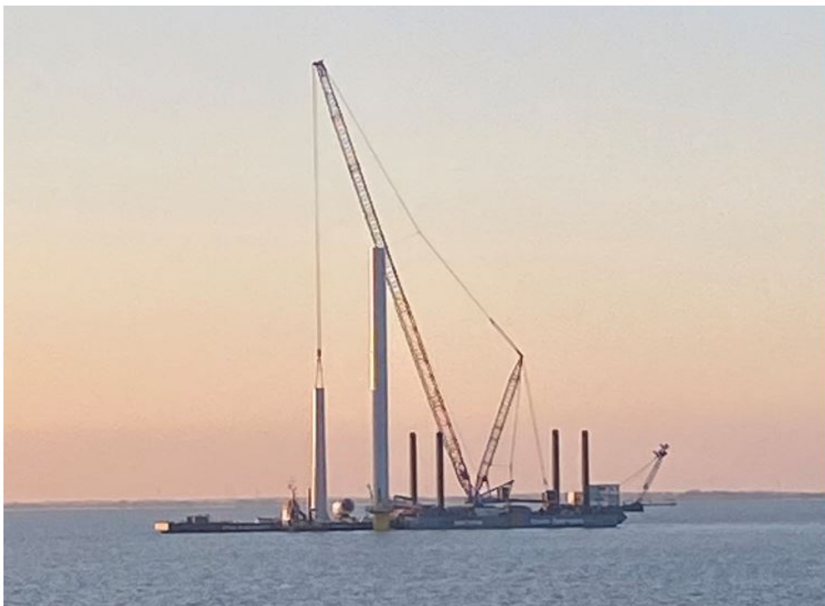
Figure 10: Side view of the CAB with the long boom of 126m during the installation of the tower sections.
