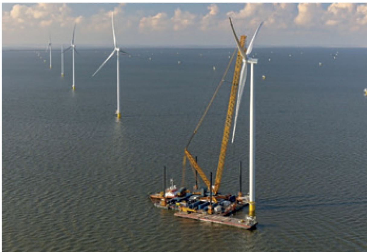
Figure 11: Top view of the CAB with the long boom of 126m during the installation of the blades.
