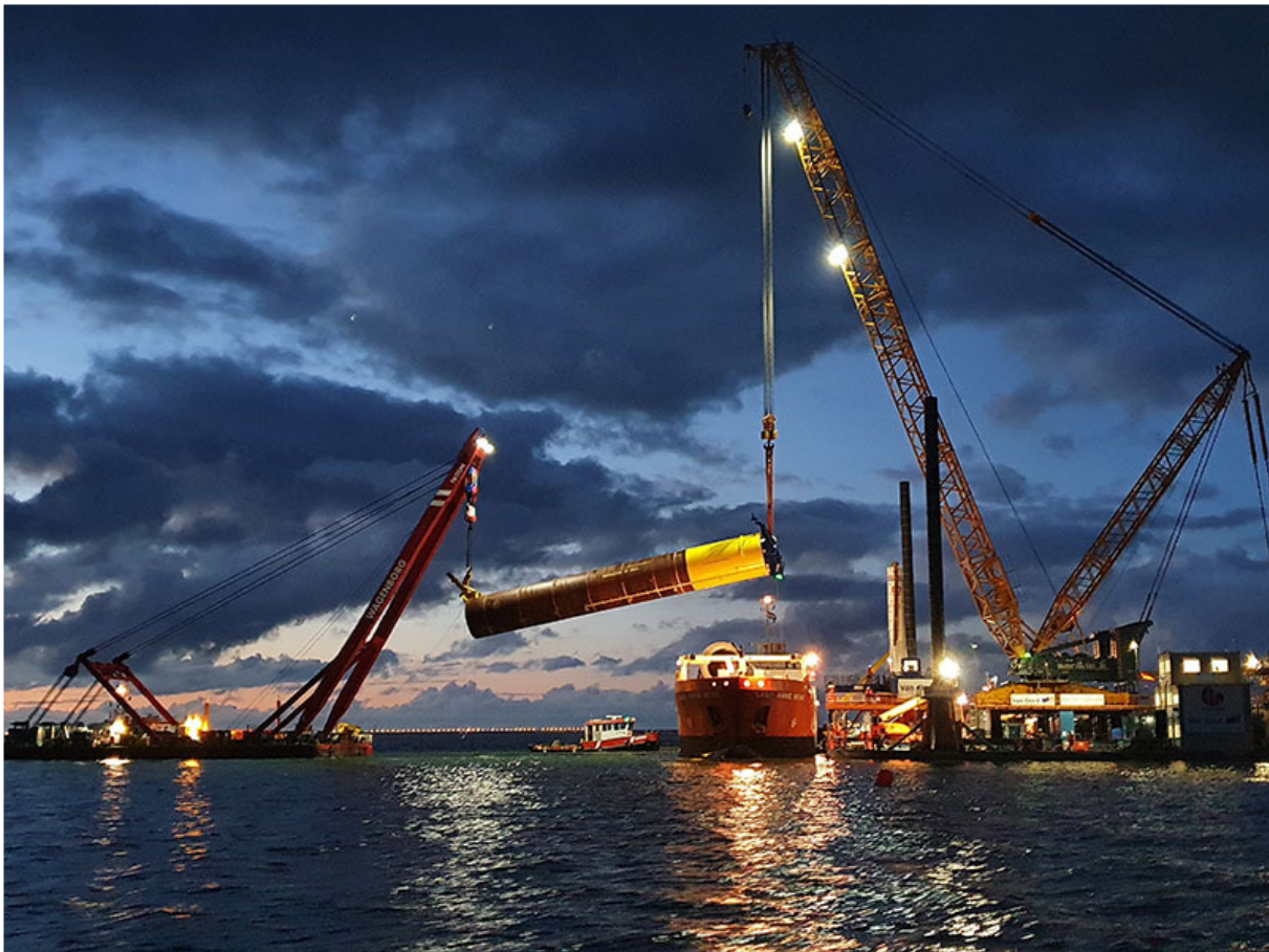
Figure 7: Side view of the CAB plus a floating sheerleg crane during the tilting up of a the monopile.
