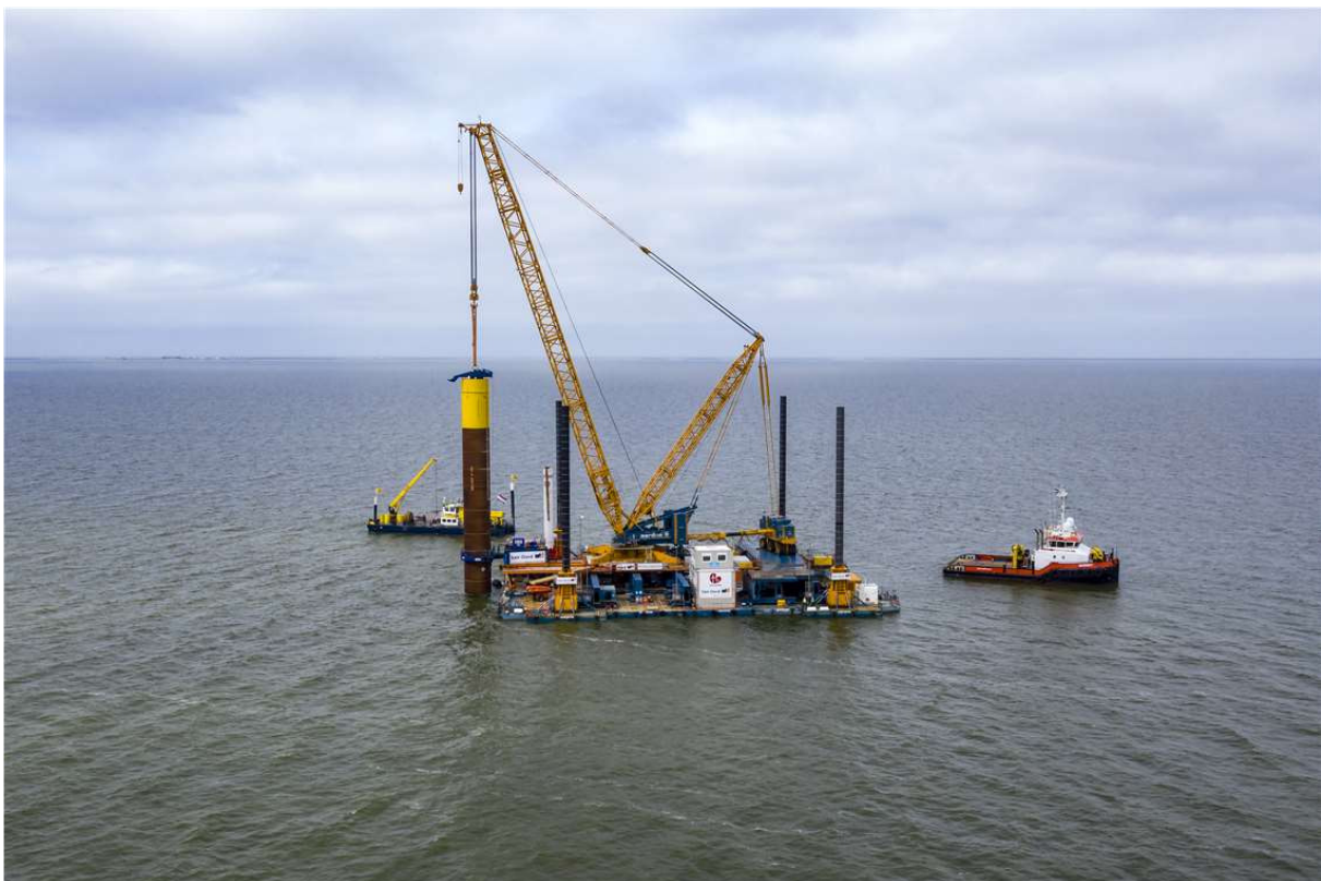
Figure 8: Side view of the CAB during the installation of a monopile on its final lake place.
