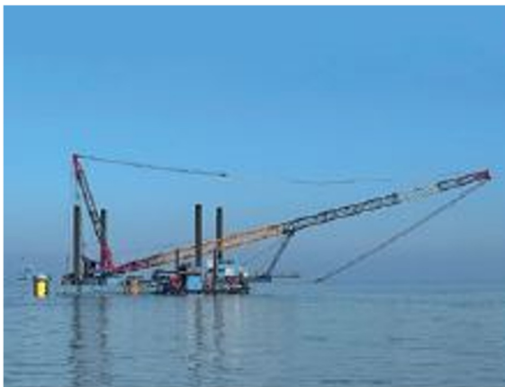
Figure 5: Specific fastening system of the 115 meters boom during the transits among different towers.
