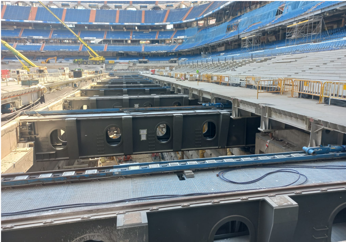
Figure 17: Skidding the Hypogeum Top Slab below the lateral seats.
