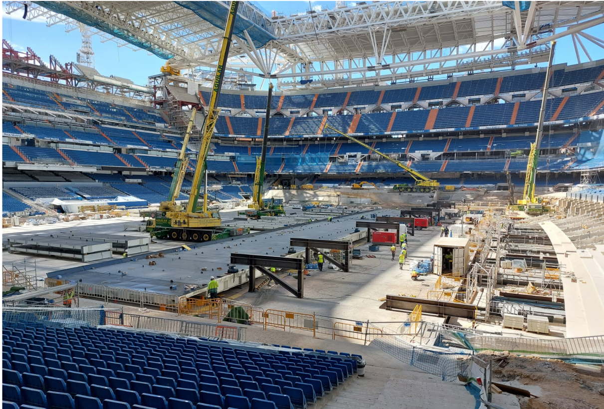
Figure 7: Hypogeum Top Slab before initial jacking.
