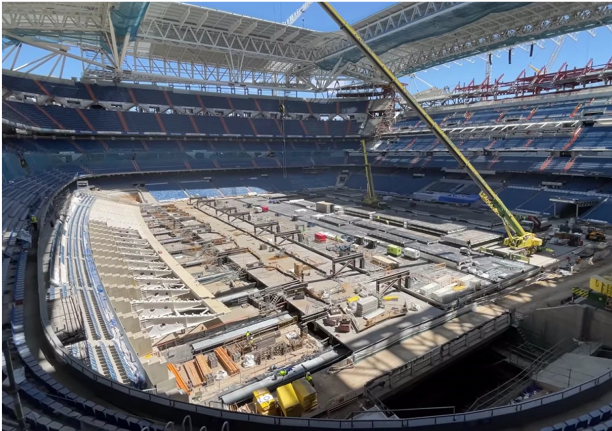
Figure 15: General top view with the Hypogeum Top Slab ready to be skidded after jacking 1,5m.
