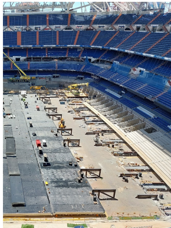
Figure 8: Hypogeum Top Slab before initial jacking.
