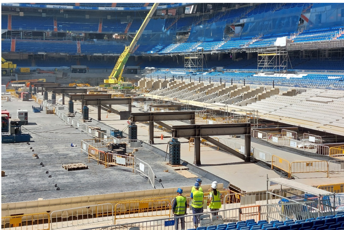
Figure 14: Eight cantilever gantries with 250t climbing jacks after jacking 1,5m the Hypogeum Top Slab.
