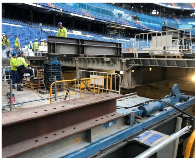
Figure 10: Cantilever beams with 250t climbing jacks
