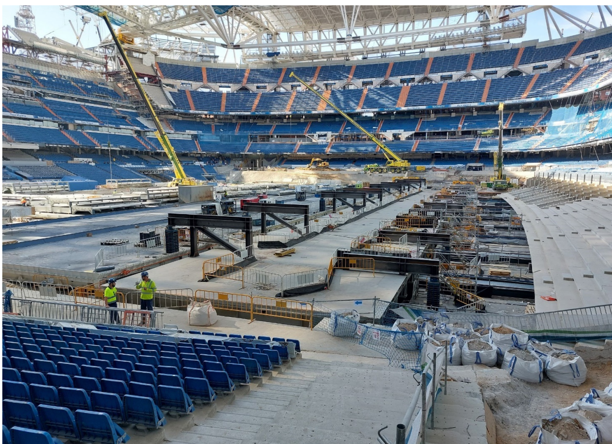
Figure 13: Hypogeum Top Slab after 1,5m jacking.
