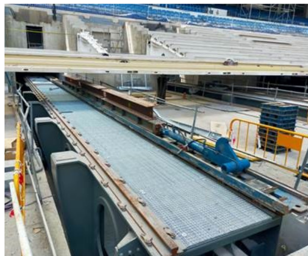
Figure 11: Skidding lines on the retractable beams.
