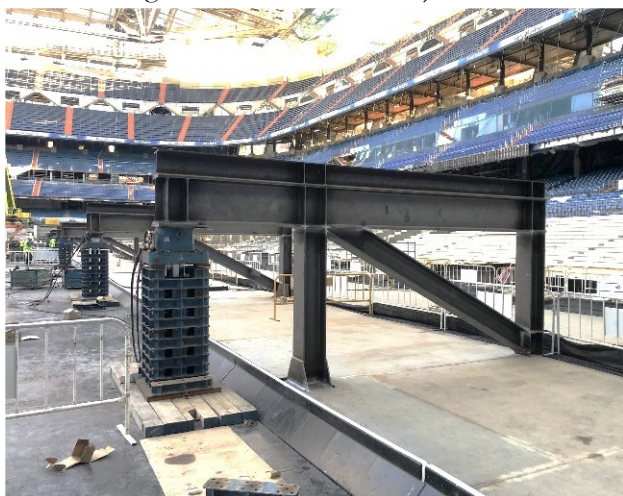
Figure 9: Cantilever gantries with 250t climbing jacks
