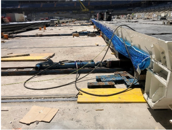
Figure 12: Push-pull units moving the tray n°6.
