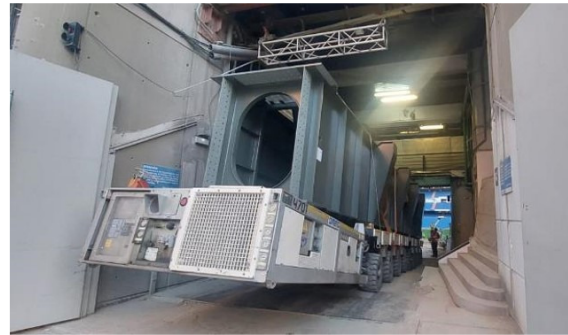
Figure 2: Retractable steel beam passing through the internal stadium gates.
