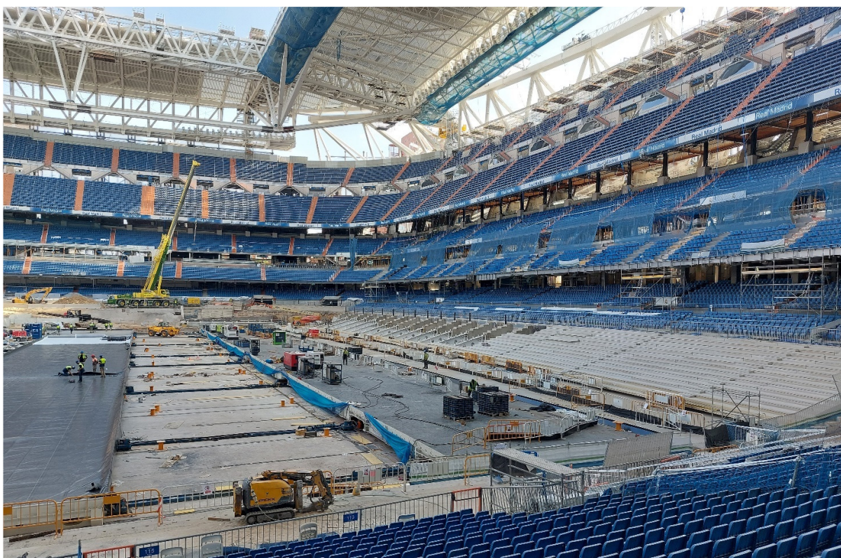
Figure 20: Grass Tray N°6 at the end of the skidding side by side the Hypogeum Top Slab.
