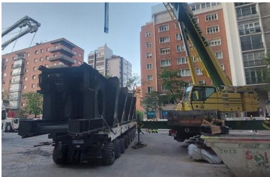
Figure 1: Retractable steel beam being loaded outside the stadium.
