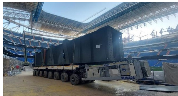
Figure 4: Retractable steel beam inside the stadium driving to the Hypogeum.
