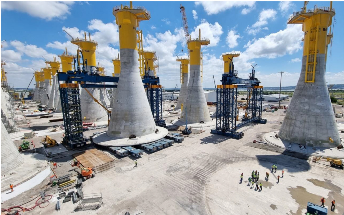
Figure 10: GBS transferred from the gantry to the SPMTs. Outside part of the gantry removed to start the transport
