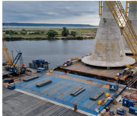
Figure 1: Spanning steel platform 11,8m length.
