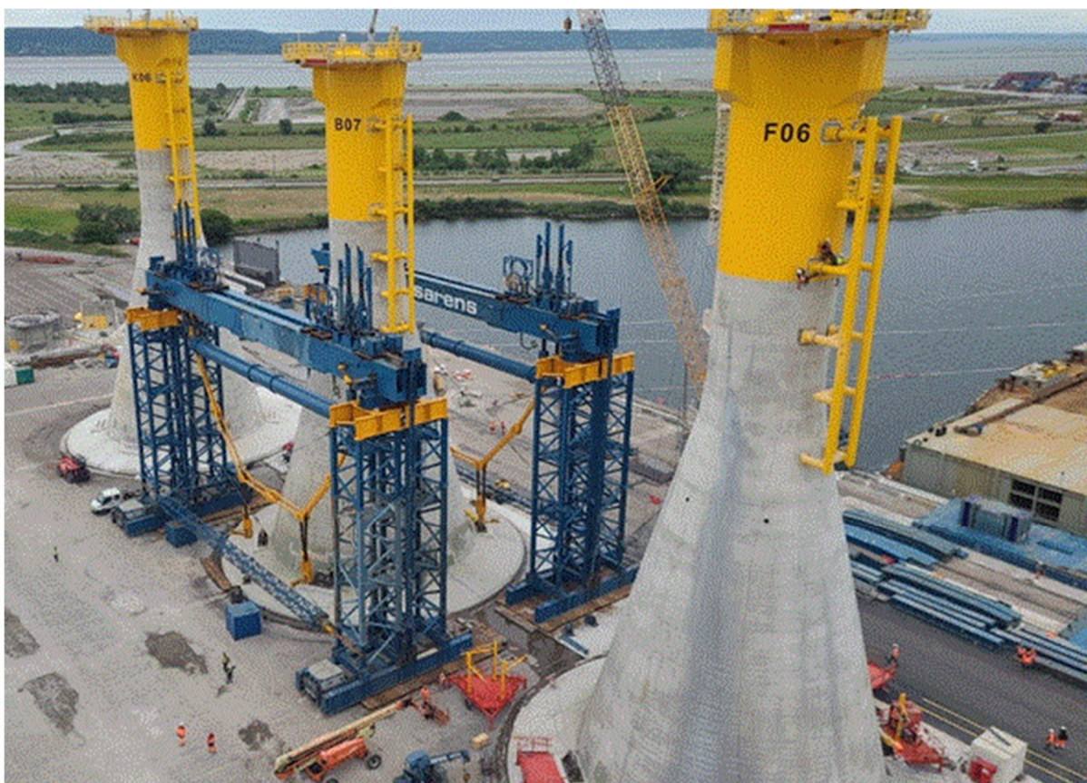
Figure 8: Top view of the lifting gantry ready to lift a GBS.
