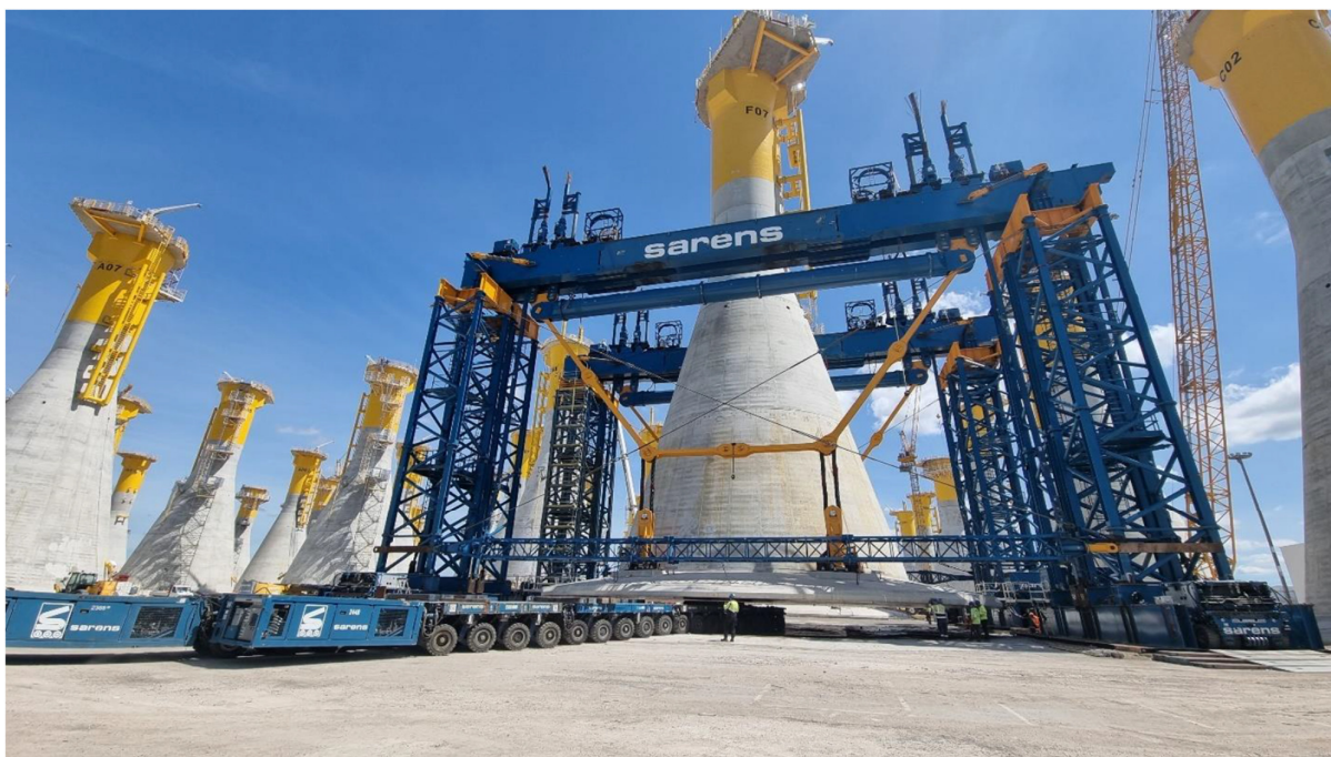
Figure 9: GBS already lifted and held on the gantry while the SPMTs drive below it.
