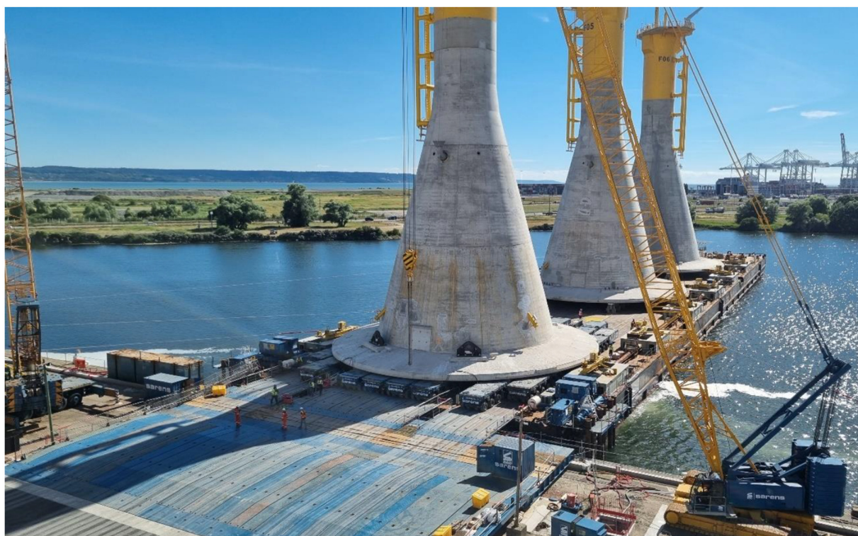
Figure 13: Last GBS loaded out in the cargo Barge, ready to be transferred to the deck grillage.
