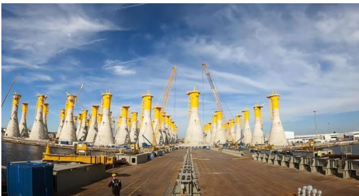
Figure 7: General view from the bow of the cargo barge before starting the load out of the GBS.
