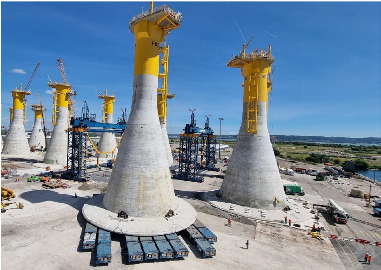
Figure 11: GBS driving from its fabrication place to the quay.
