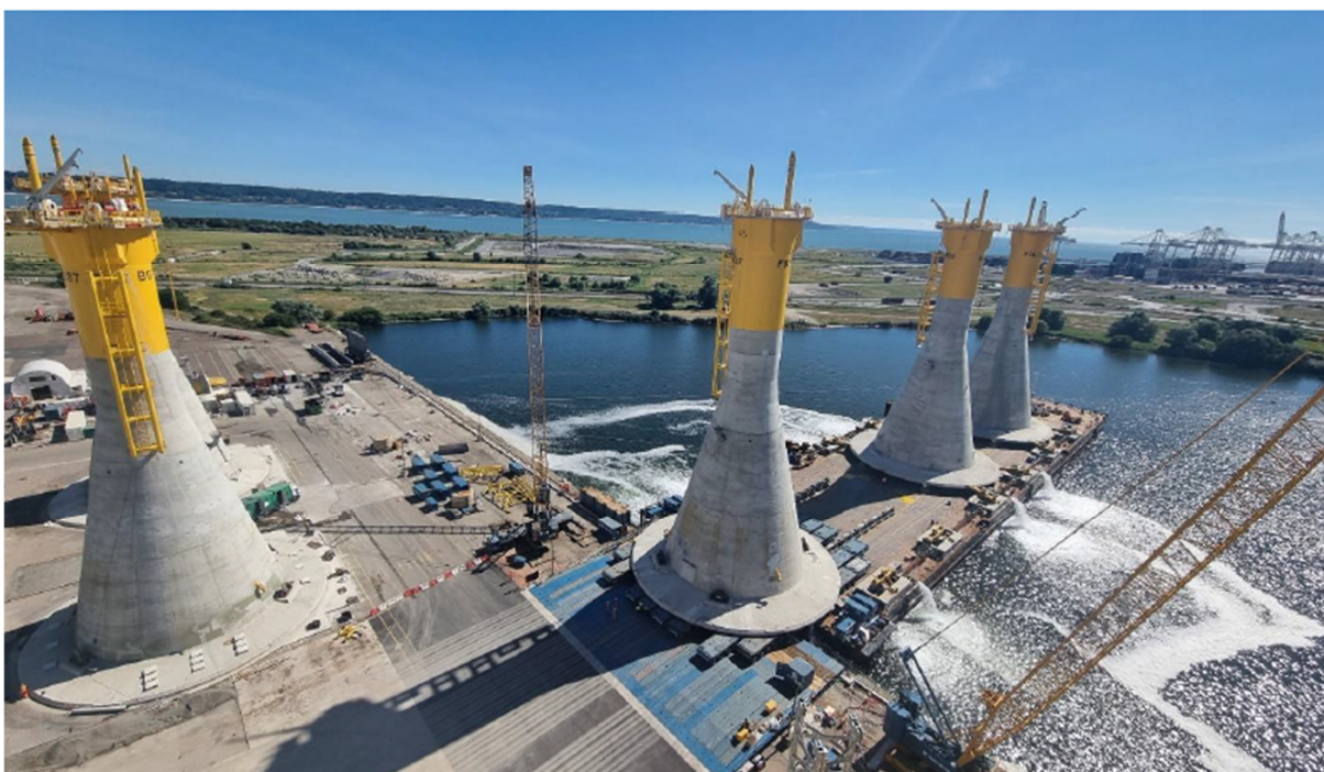
Figure 12: Top view of the last GBS to be loaded out in the cargo barge. External ballasting system in operation.
