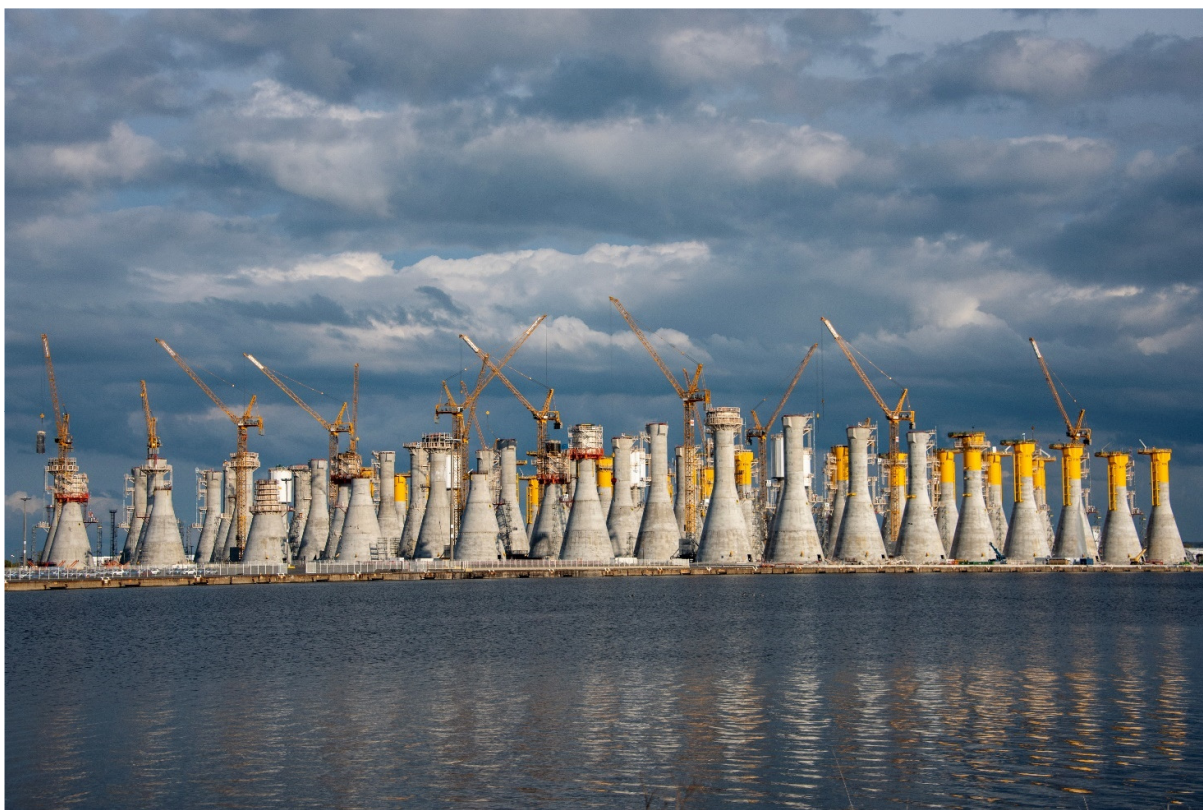
Figure 6: General view from the water of the 71 x 5.000 tons GBS at port of Le Havre.
