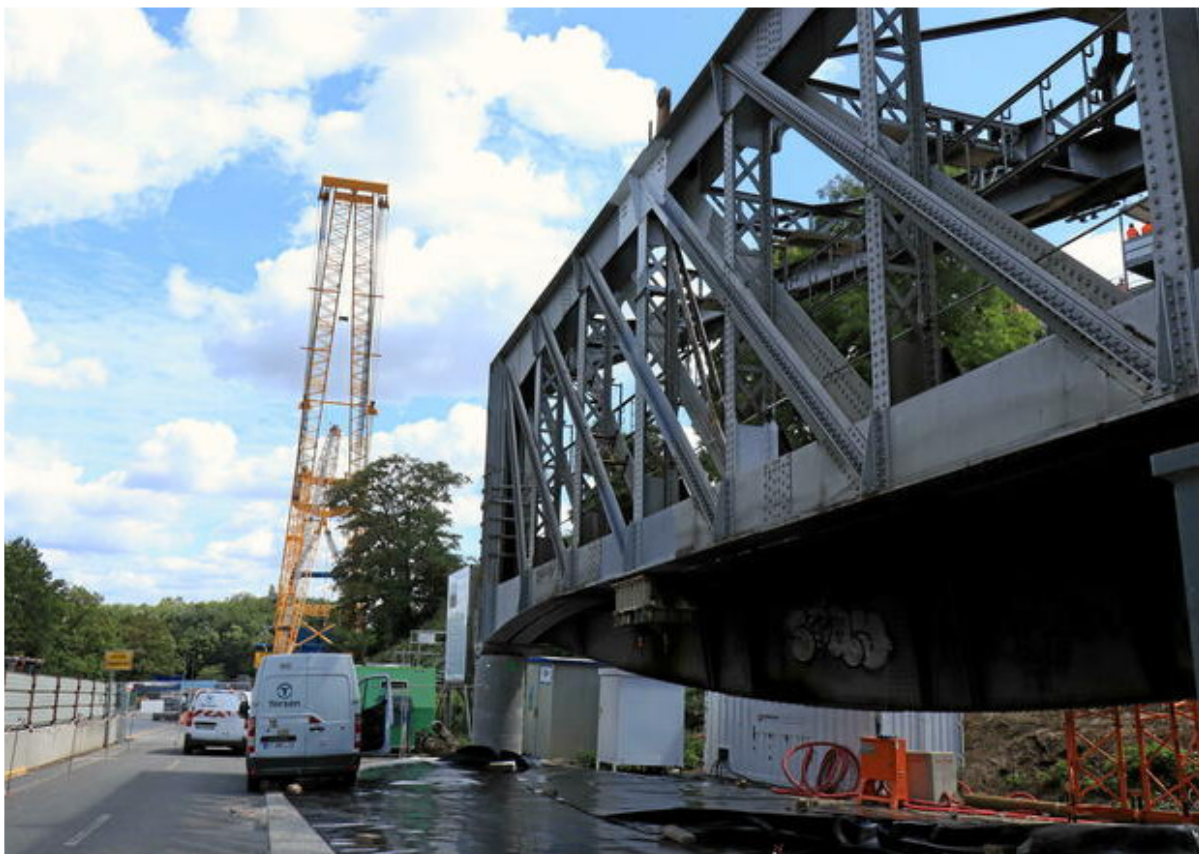
Figure 14: Old Gallardon bridge in demolition area
