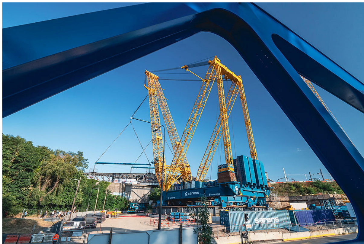
Figure 11: Lifting of old Chartres bridge seeing from Gallardon fabrication site place
