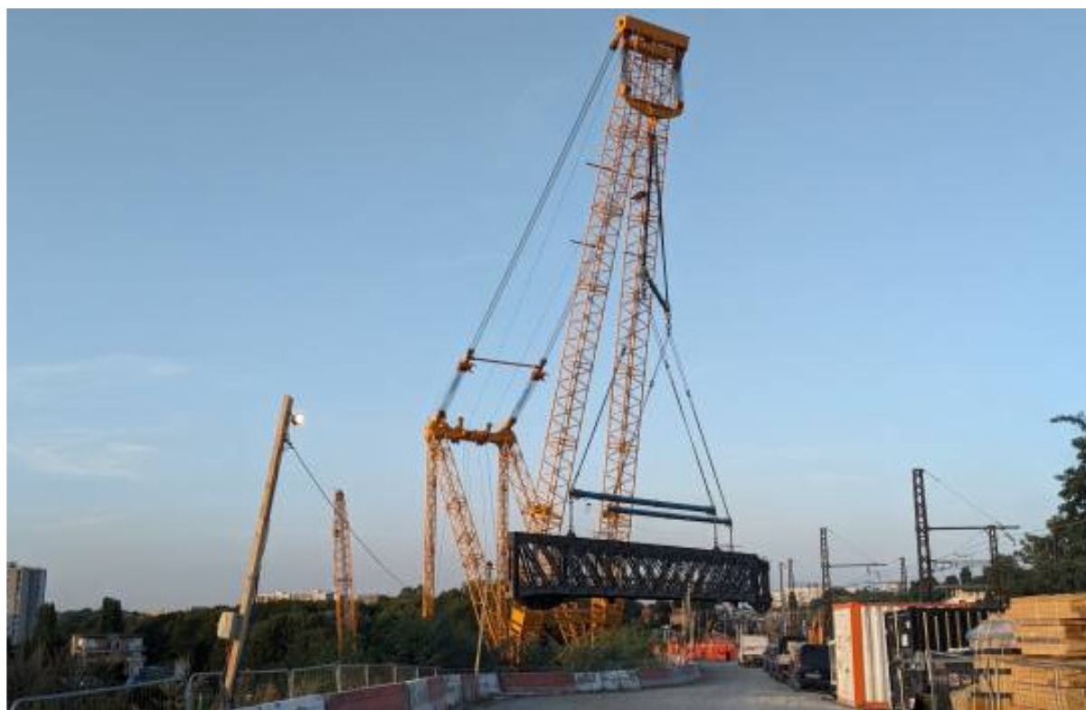
Figure 12: Lifting of old Chartres bridge
