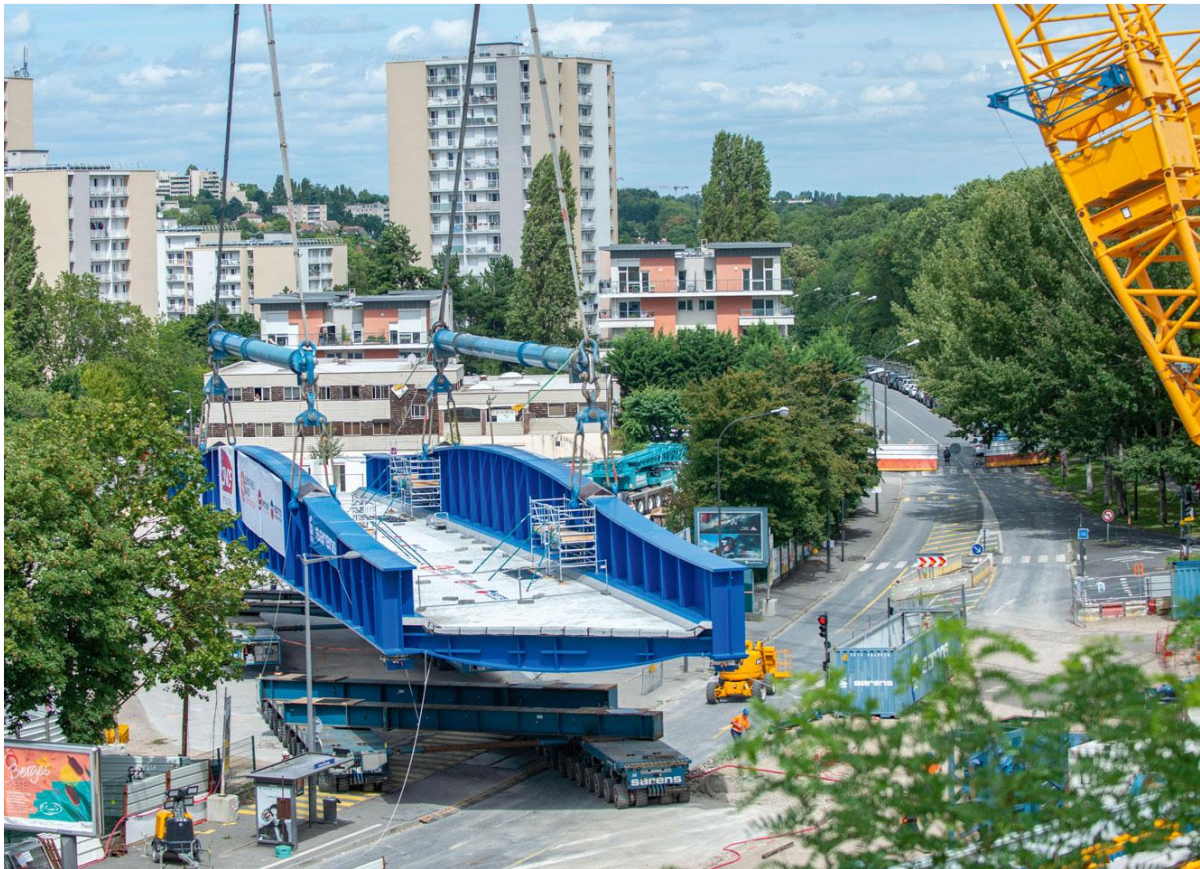
Figure 15: New Chartres bridge placed on SPMTs
