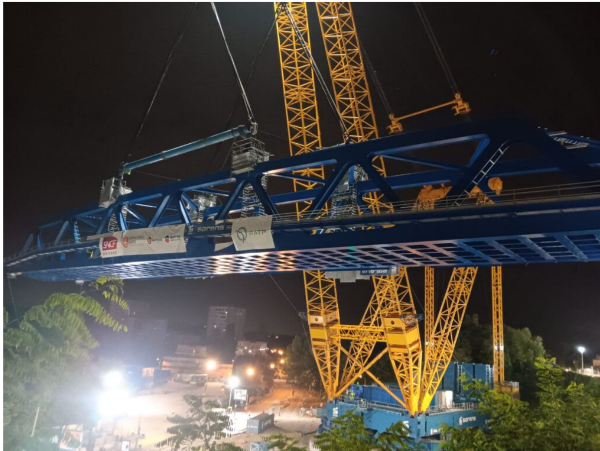
17: Lifting of new Gallardon Bridge
