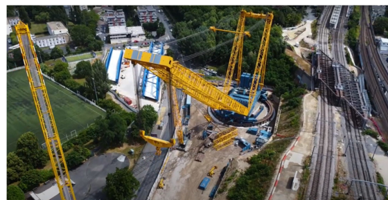
Figure 4: Aerial view of SGC-90 assembled on site
