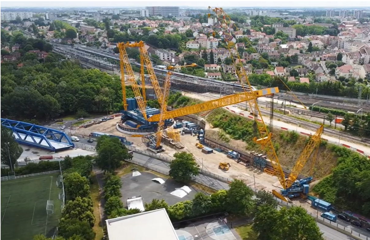
Figure 10: SGC-90 ready to lift
