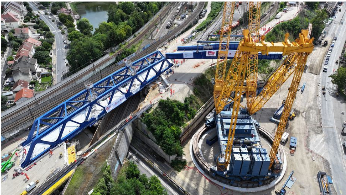
Figure 16: Lifting of new Chartres bridge
