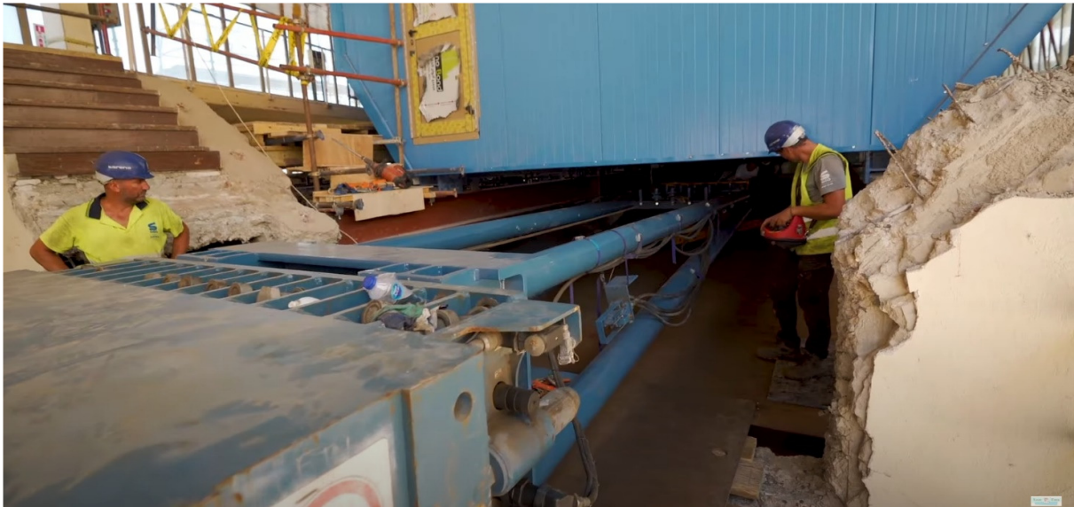
Picture 7: Installation of temporary bridge under solar boat sarcophagus using SPMTs
