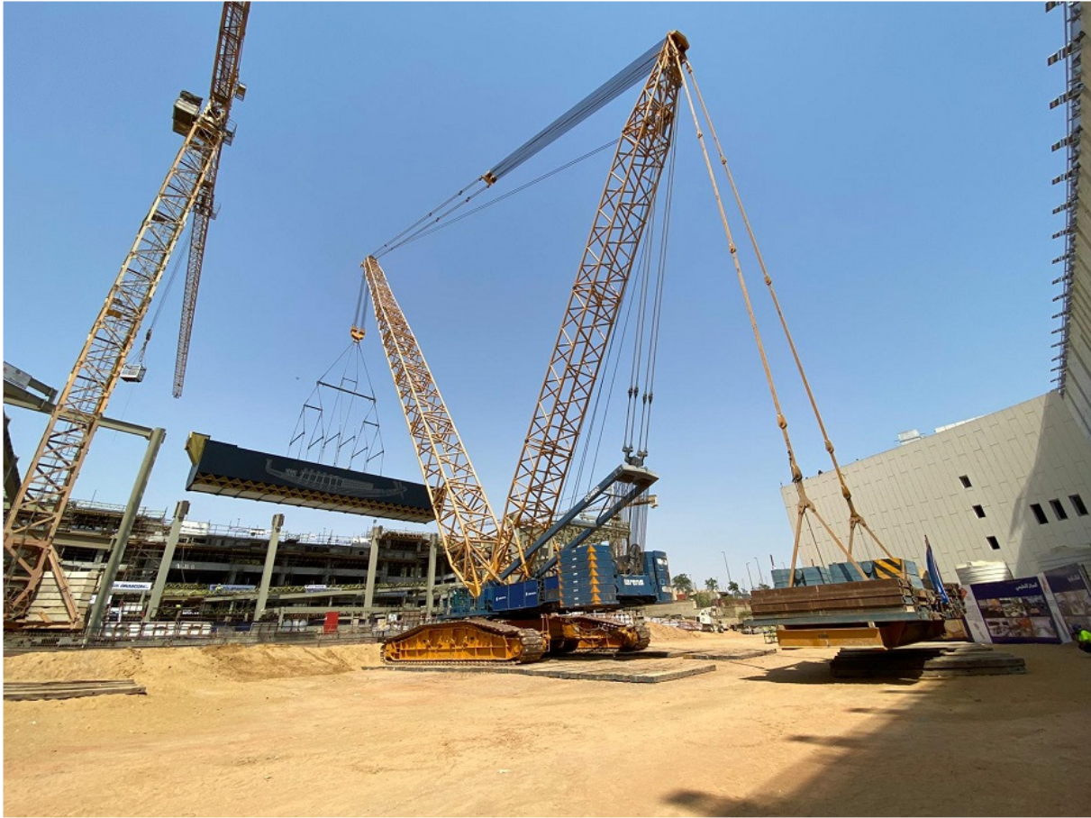
Picture 11: Lifting operation inside new dedicated museum within GEM complex
