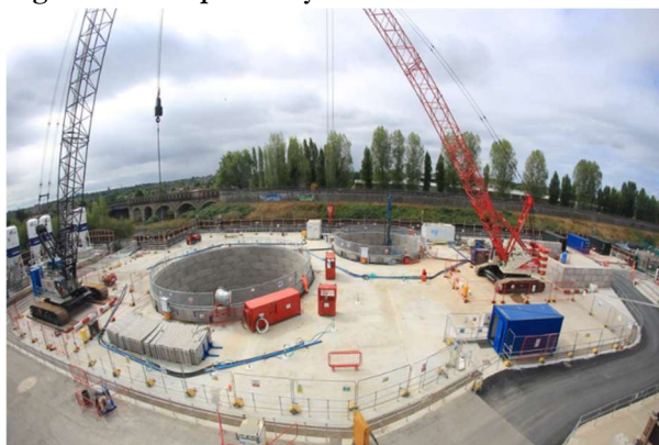
Figura 6. Greenpark Way. Pozos principal y satélite
