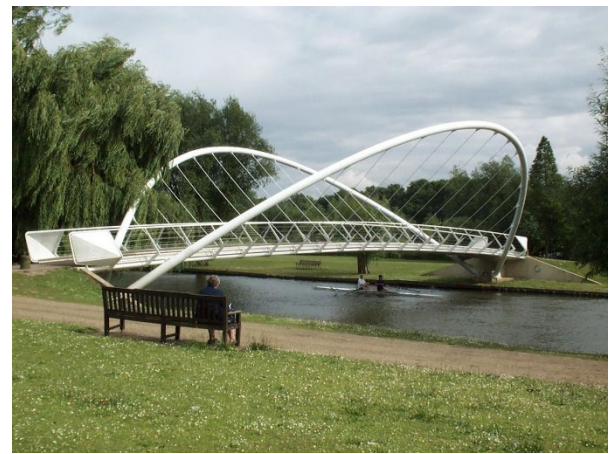
Figura 3. Butterfly Bridge, Bedford (UK) www.structurae.de .
