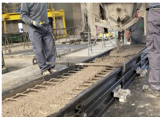
Fig. 2. View of the specimen during concreting
