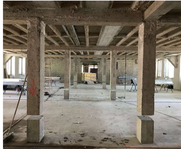
Figure 5: Columns cut during the construction.
