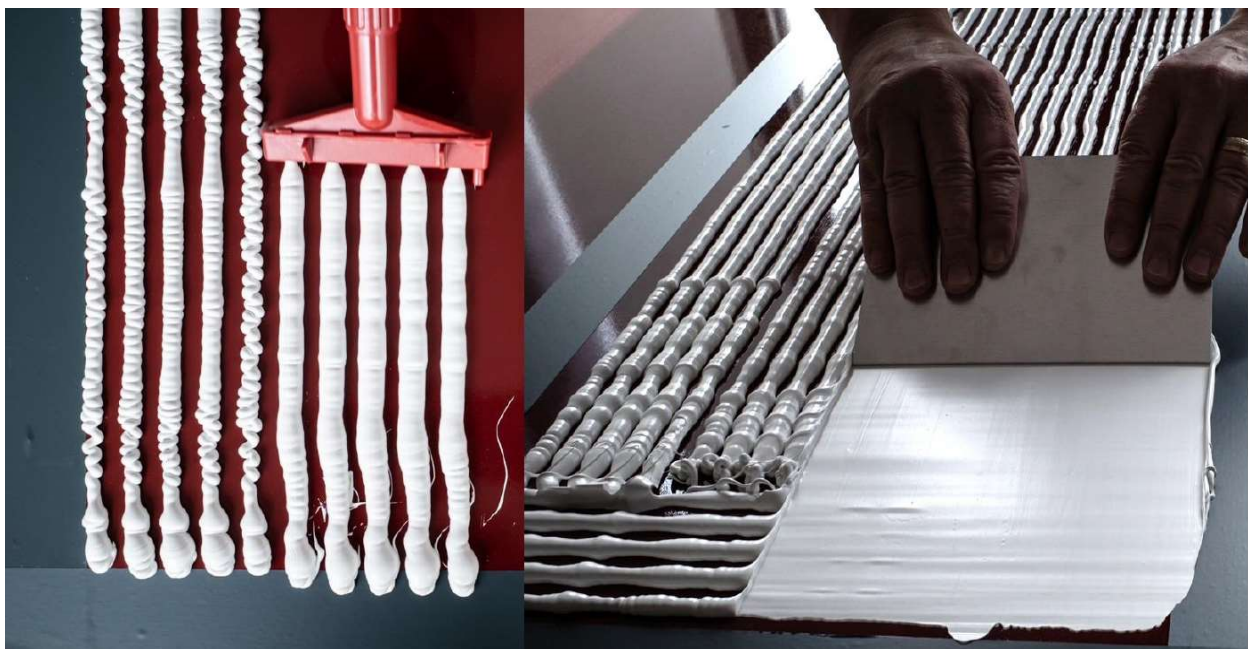
Figure 11 Application of the silicon layer on the existing spandrel glass panels.
