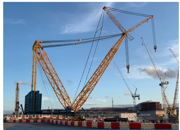
Figure 10: SGC-250 boom up ready to lift
