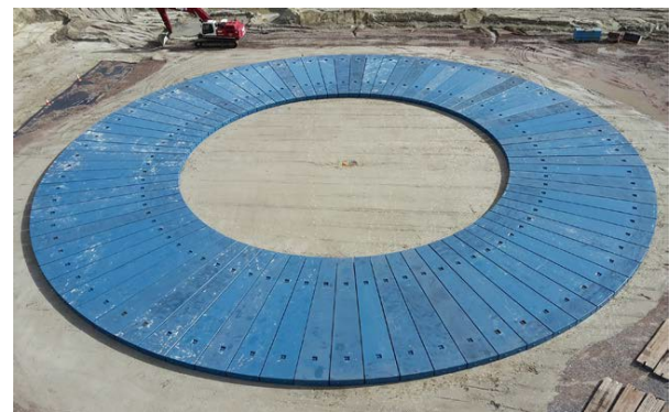
Figure 3: 52.8m OD spreader mats
