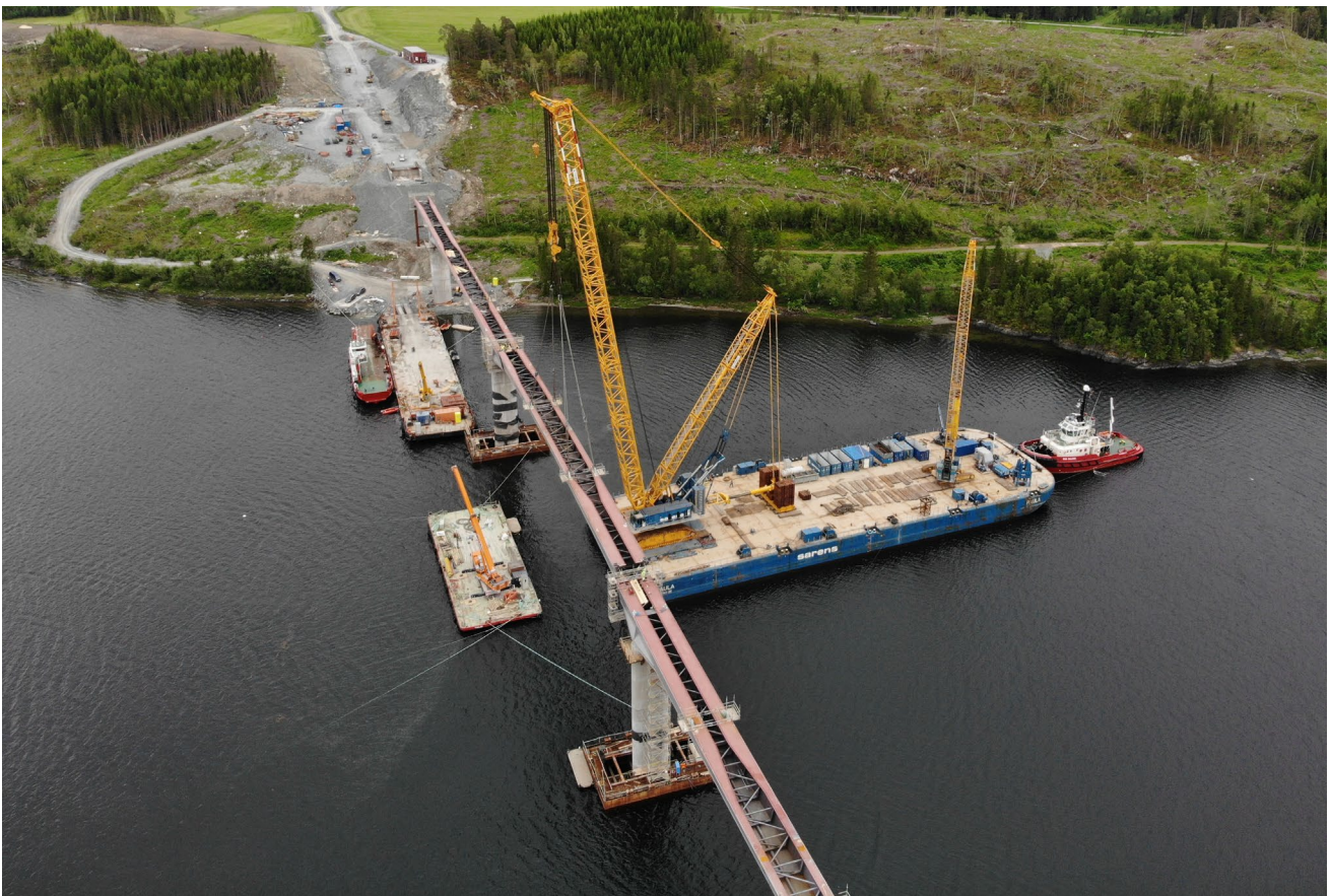
Figure 12: General view of the fourth segment installing at its final bridge position
