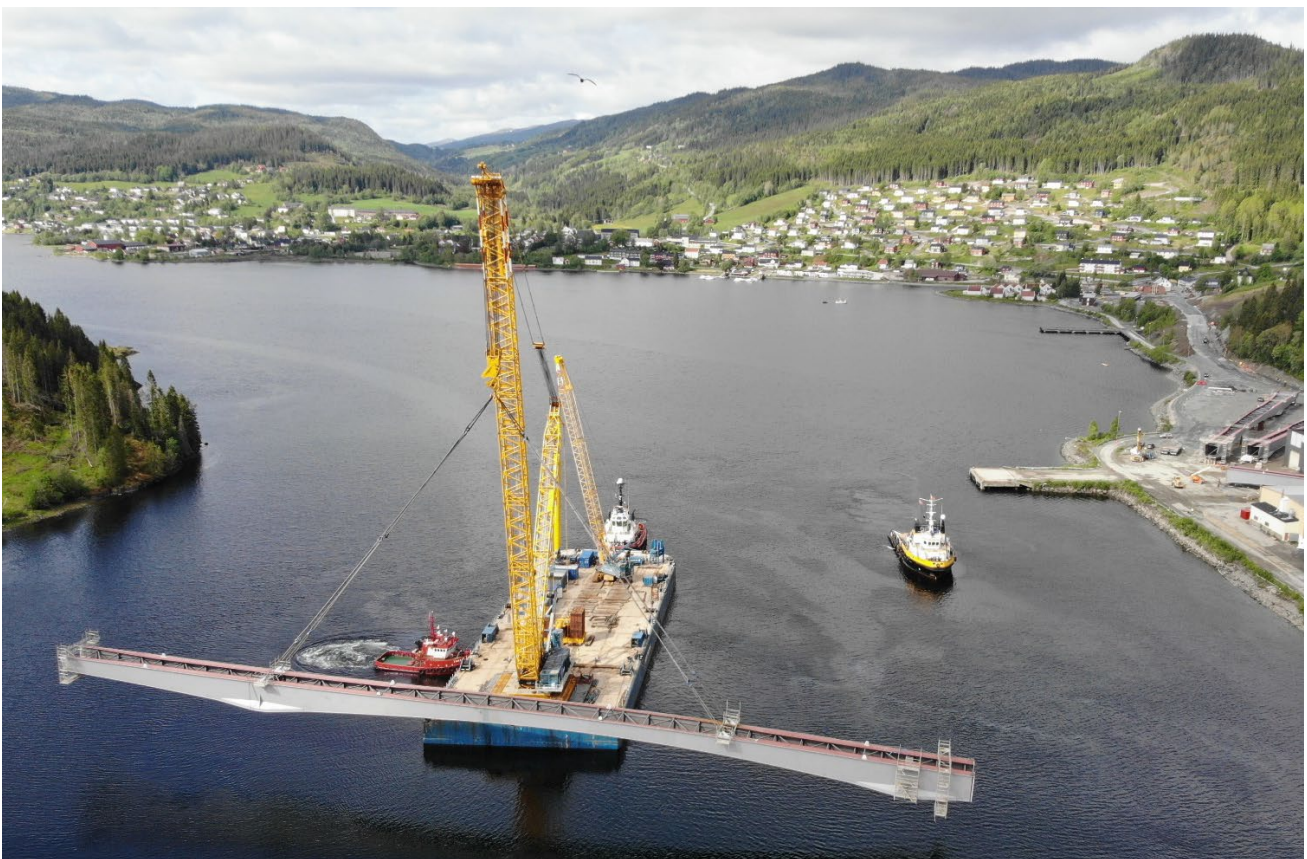
Figure 6: General view of the first segment sailing from Malm to its final bridge position
