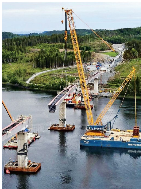
Figure 8: General view for typical installation of one segment.
