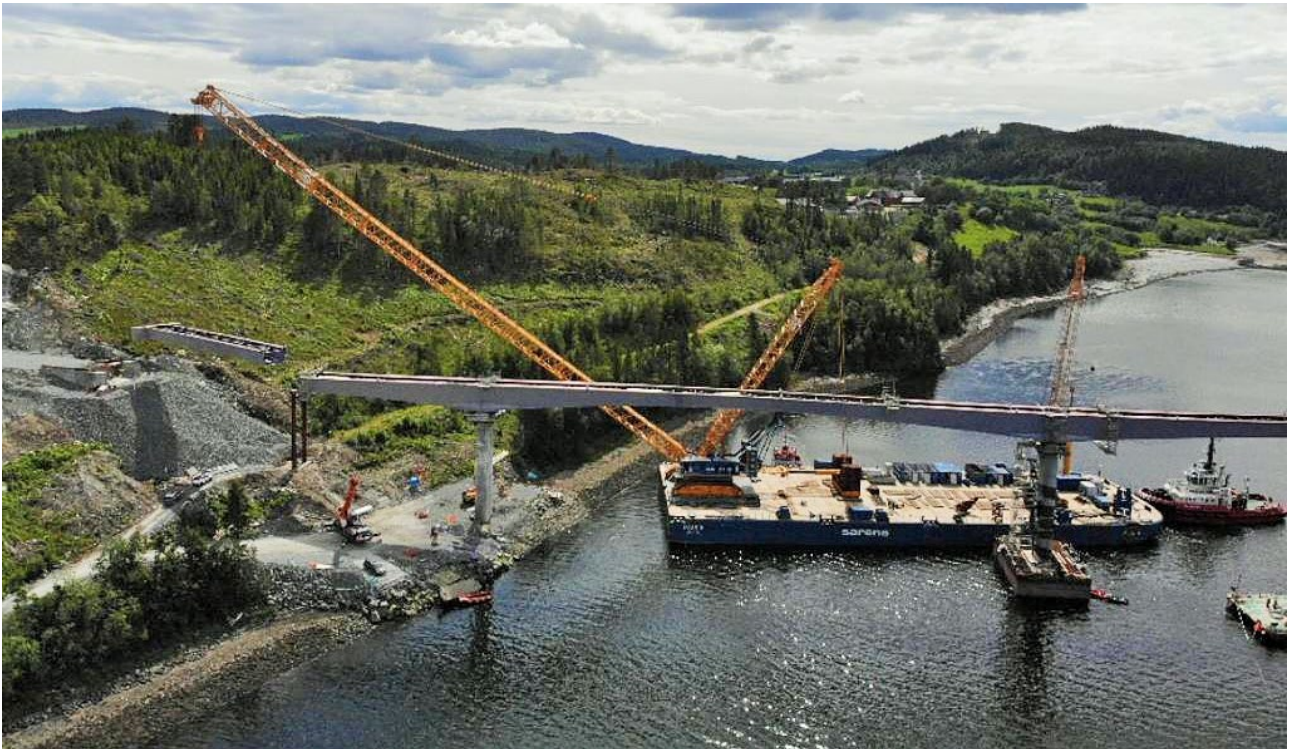
Figure 13: Installation of the fifth segment. Worst load case: SSL 120 meters main boom, 90t @ 100 m radio
