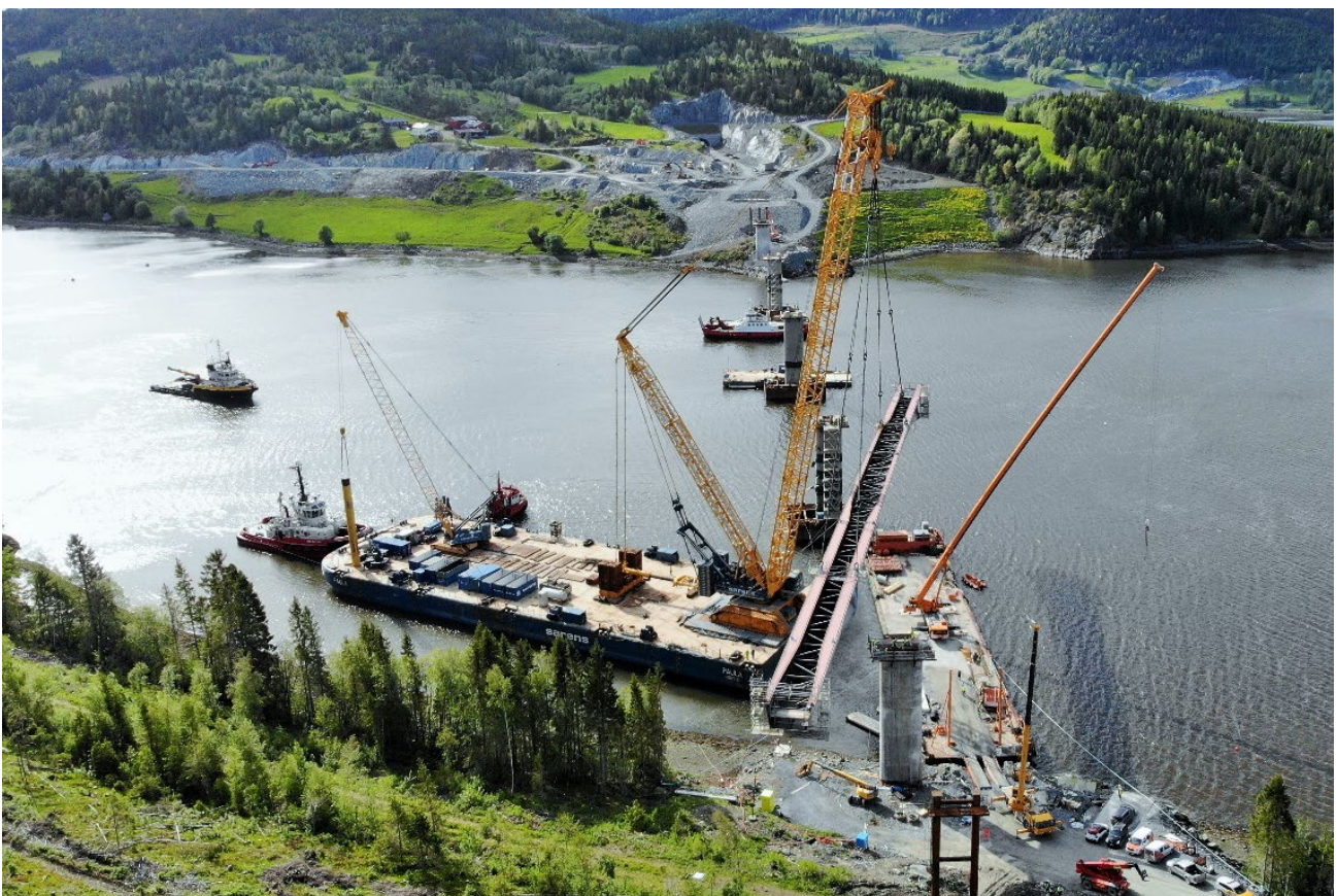
Figure 9: General view of the first segment arriving to its final bridge position
