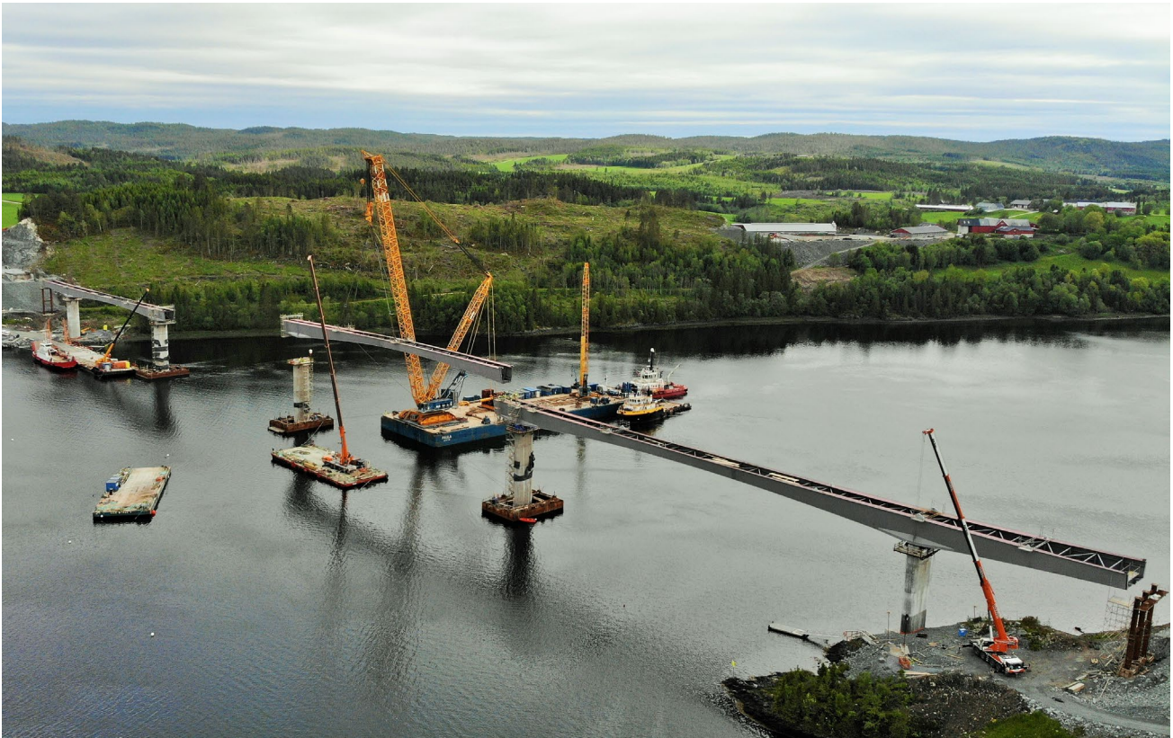
Figure 11: General view of the third segment installing at its final bridge position.
