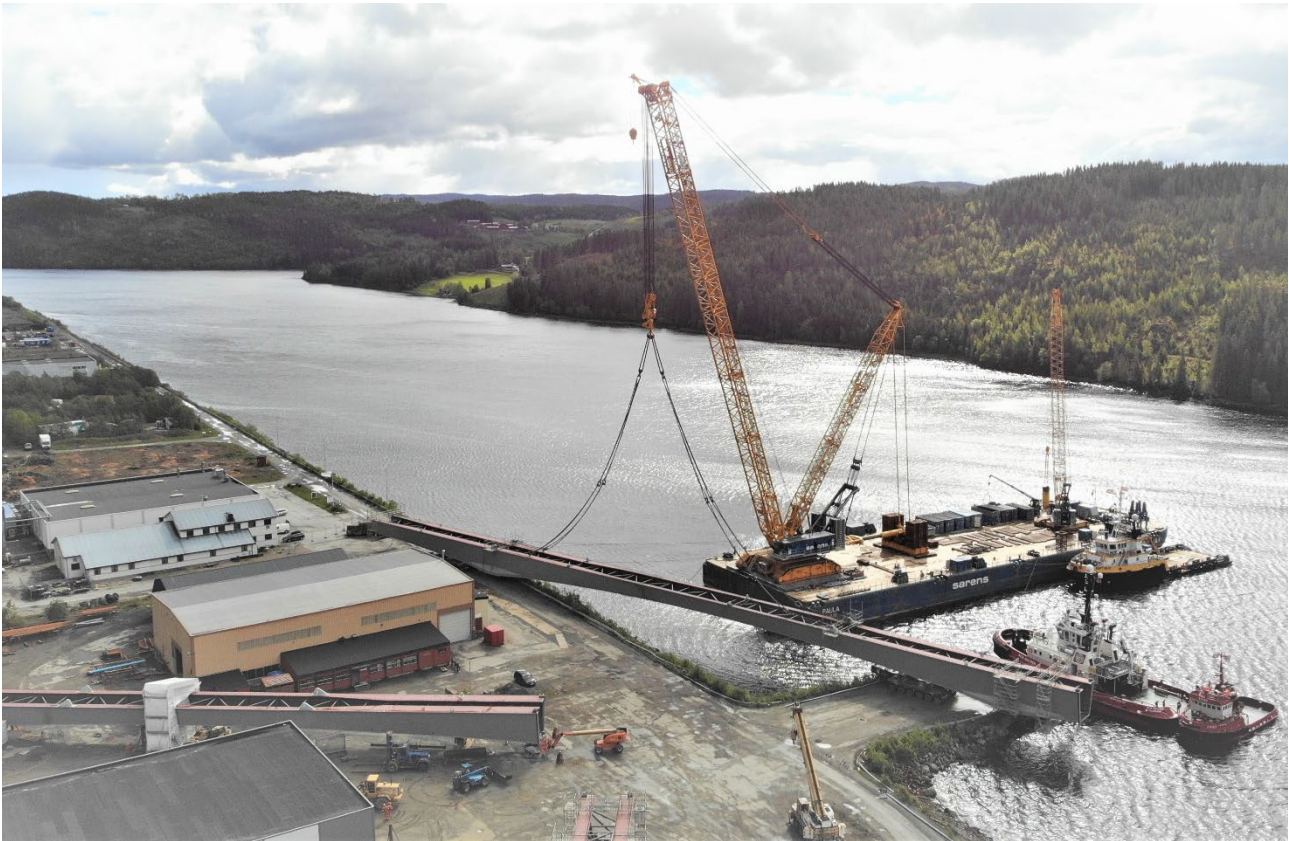
Figure 5: General view of the first segment on SPMT's brought to the reach of the CC8800 (hooking phase).
