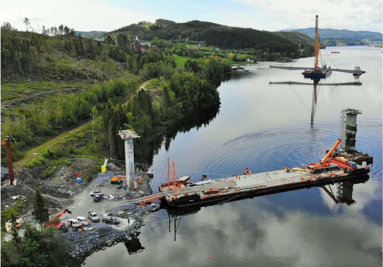
Figure 9: General view of the first segment arriving to its final bridge position
