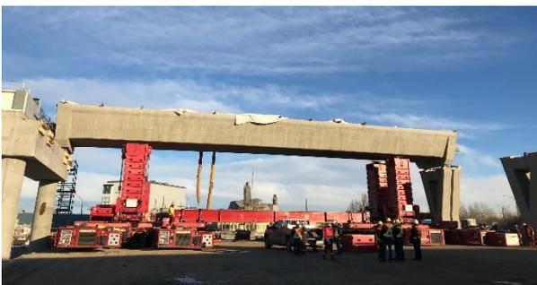
Figure 22. Erection of a single track beam.(© TransED LRT).
