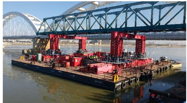
Figura 14. Carga transferida a Megajacks
