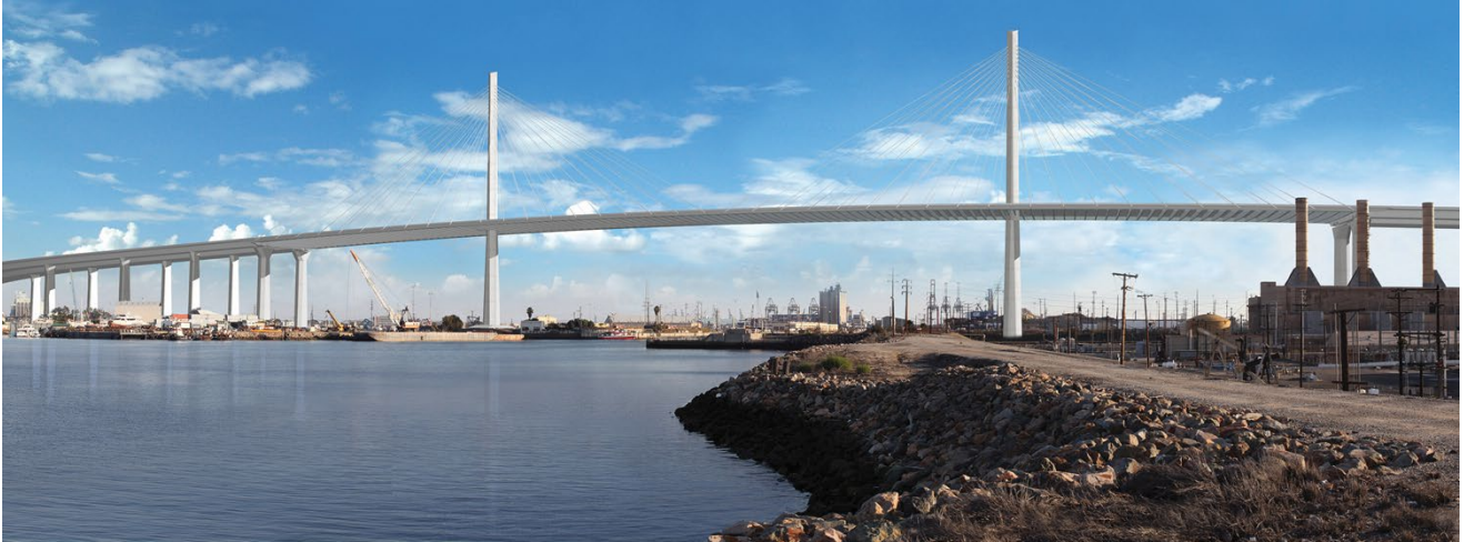
Figure 1. Rendering of Gerald Desmond Bridge Replacement Project
