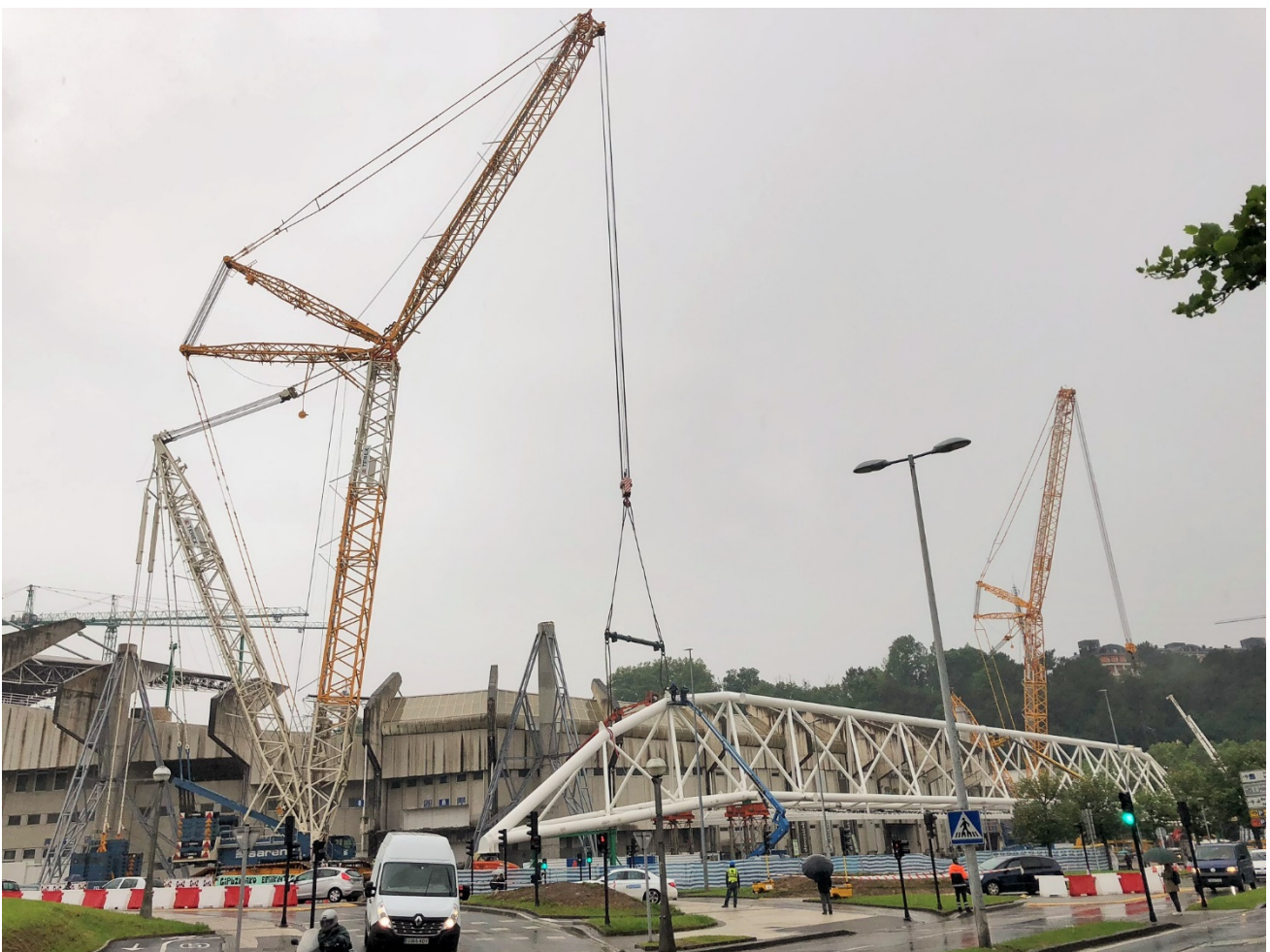
Figure 1: Initial position of the cranes for taking the load.
