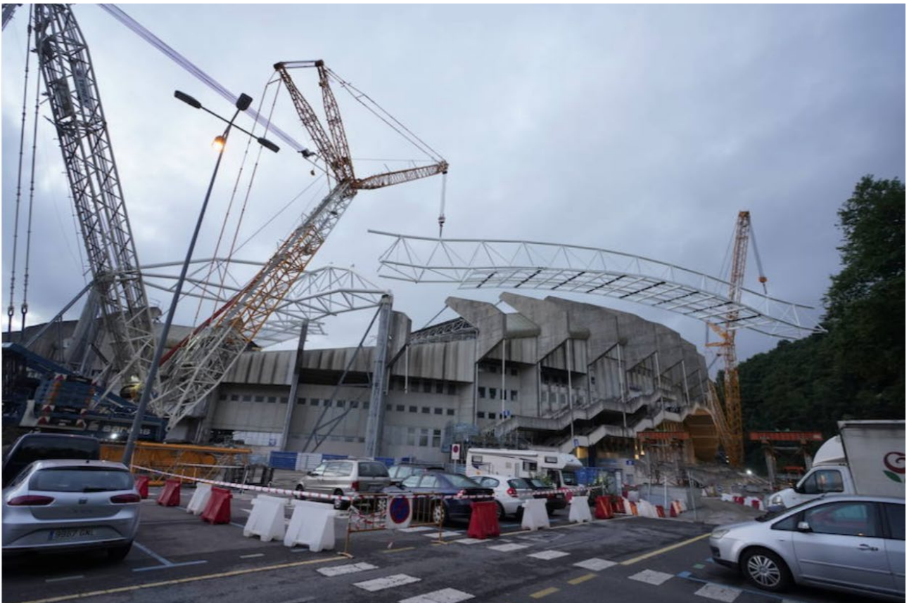
Figure 7: Intermediate position with the hook of one crane at the left already inside the stadium.
