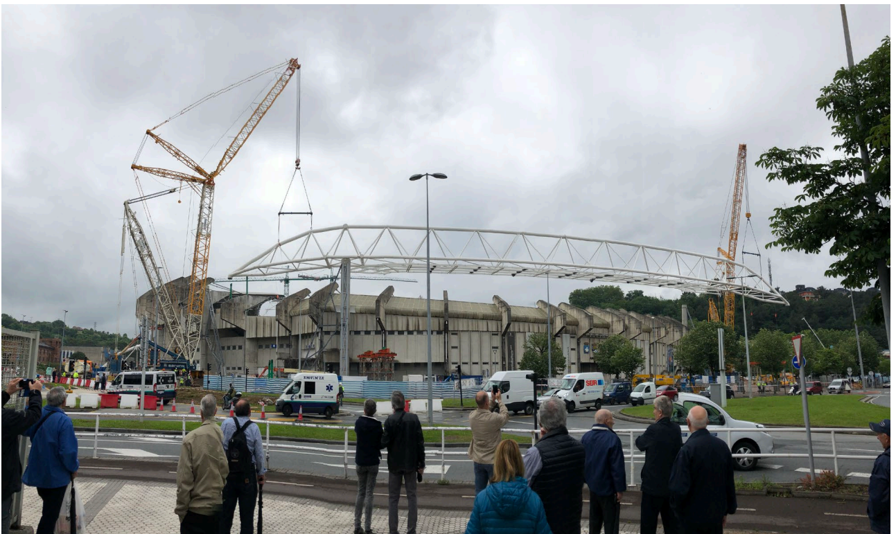
Figure 3: Intermediate position with the hook of one crane (left) already inside the stadium.
