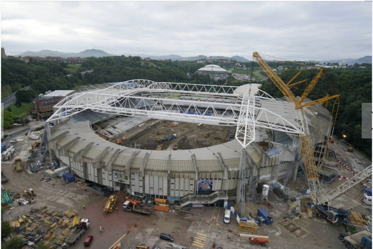
Figure 10: Final position. General view of the stadium with the 4 new trusses already installed.
