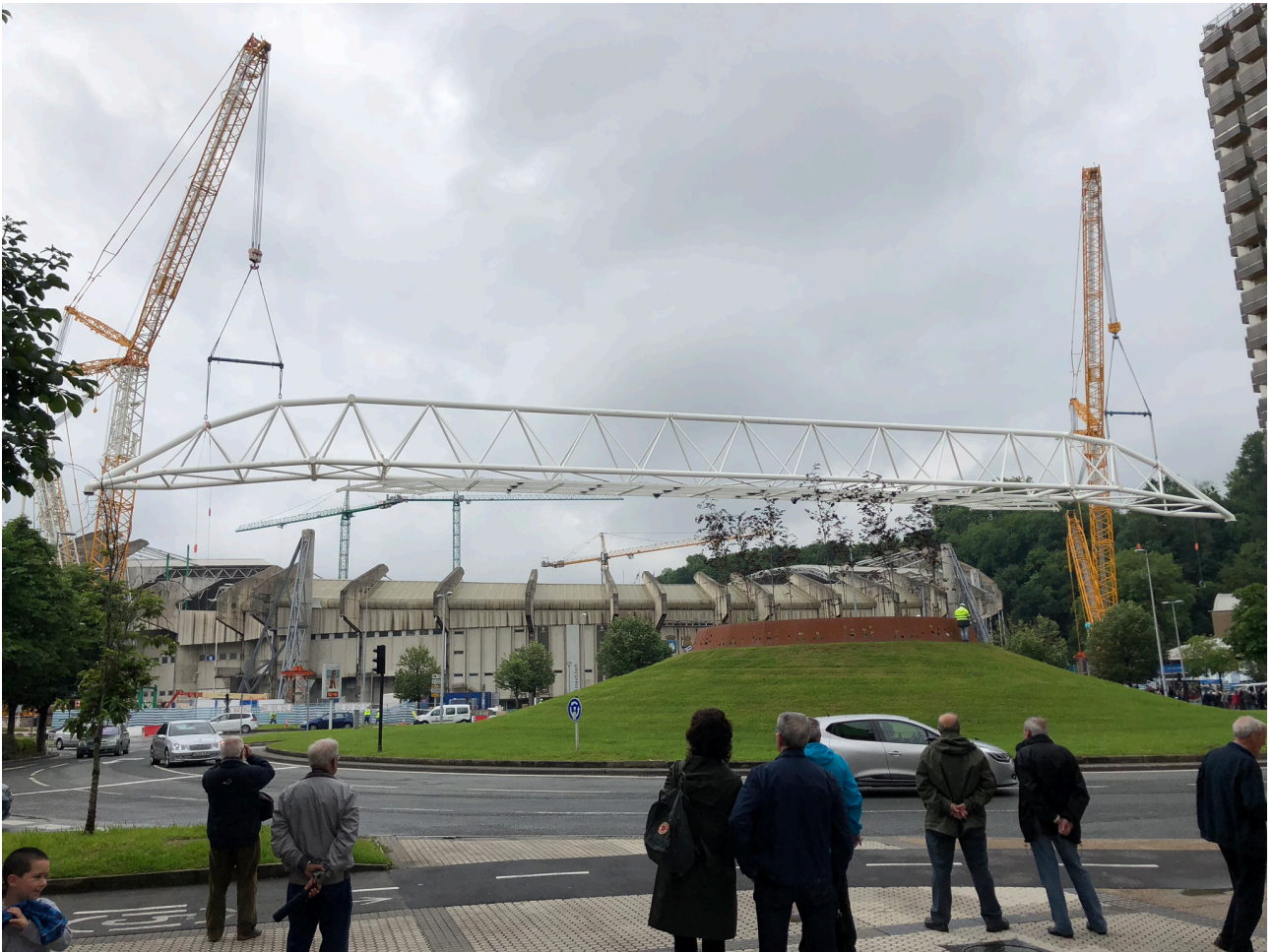
Figure 2: Intermediate position of the cranes with the truss still out site the stadium.
