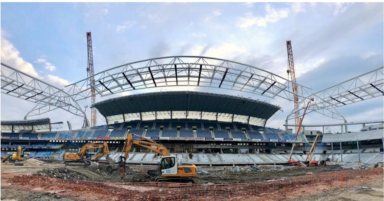
Figure 9: Inside view from the pitch right before final position. Also, visible other subcontractors working to lower the level of the pitch so the new seats over the former athletic truck can see it.
