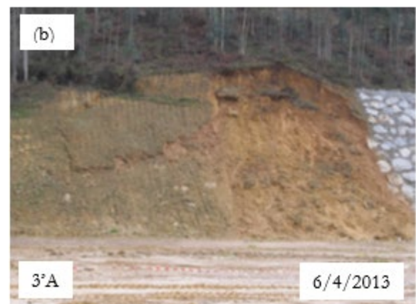
Figure 3: Landslides prior to the construction of the industrial unit. Top photo was taken on December 2010 and bottom one on April 2013.
