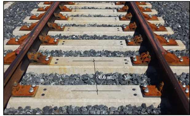
Figure 1. Usual distance between sleepers in Europe 0.6 m in High Speed and conventional ballast track.
